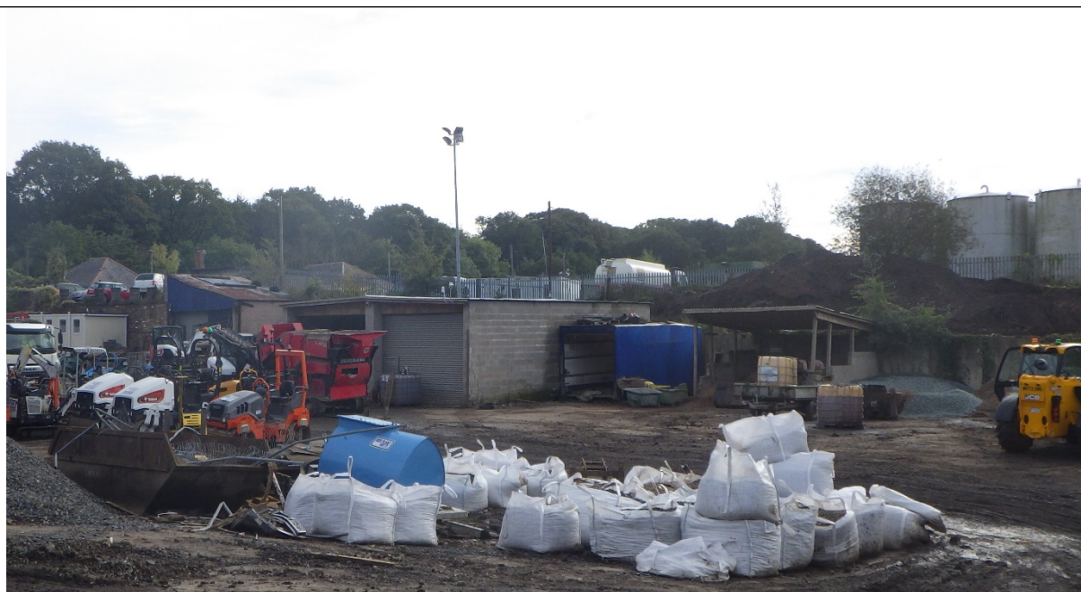
Photo showing multiple IBC on site.
