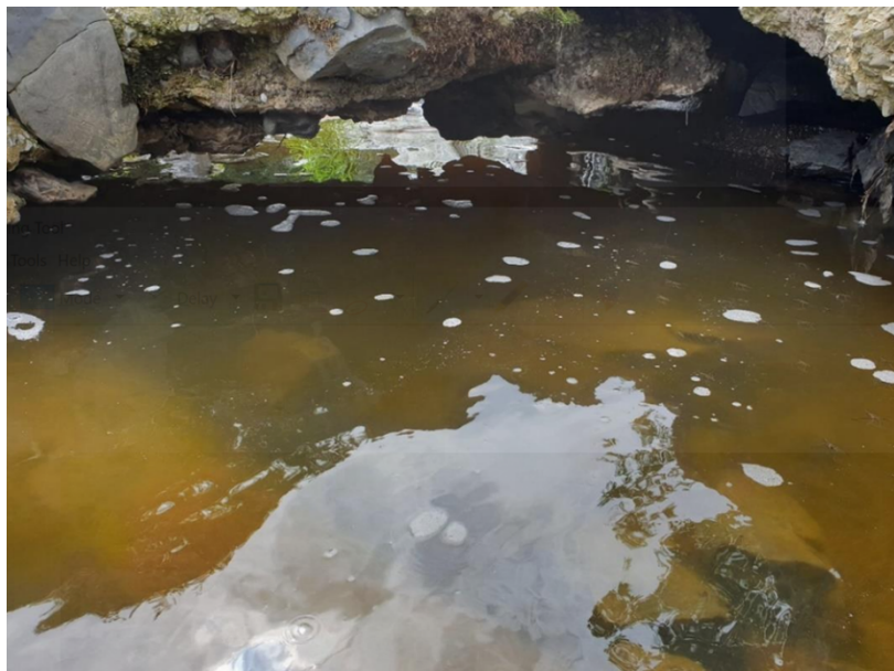
Figure 5. Evidence of undercutting under the upstream left weir channel, extracted from the WCA (August 2020).
