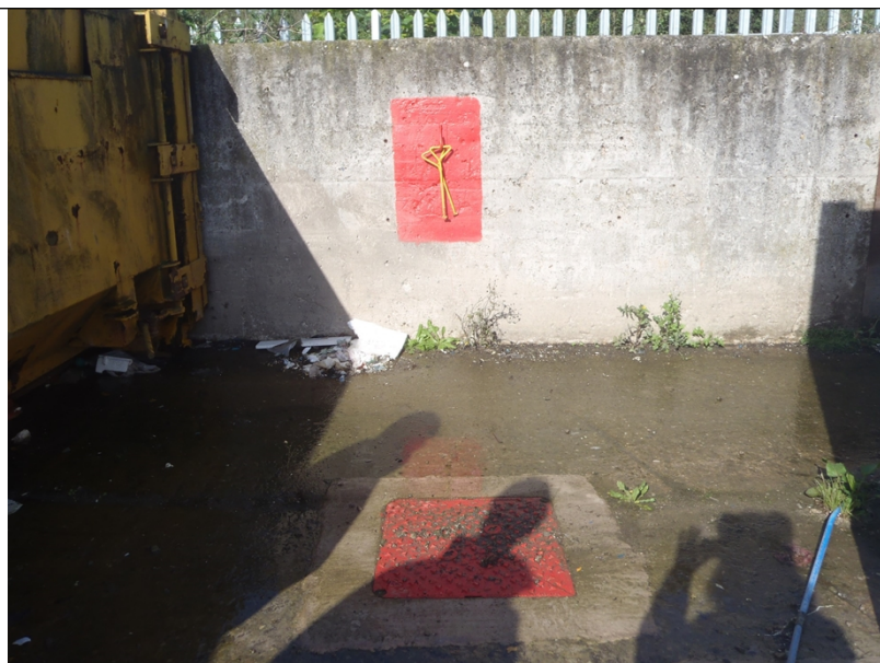
Location of stop value clearly identified and accessible
