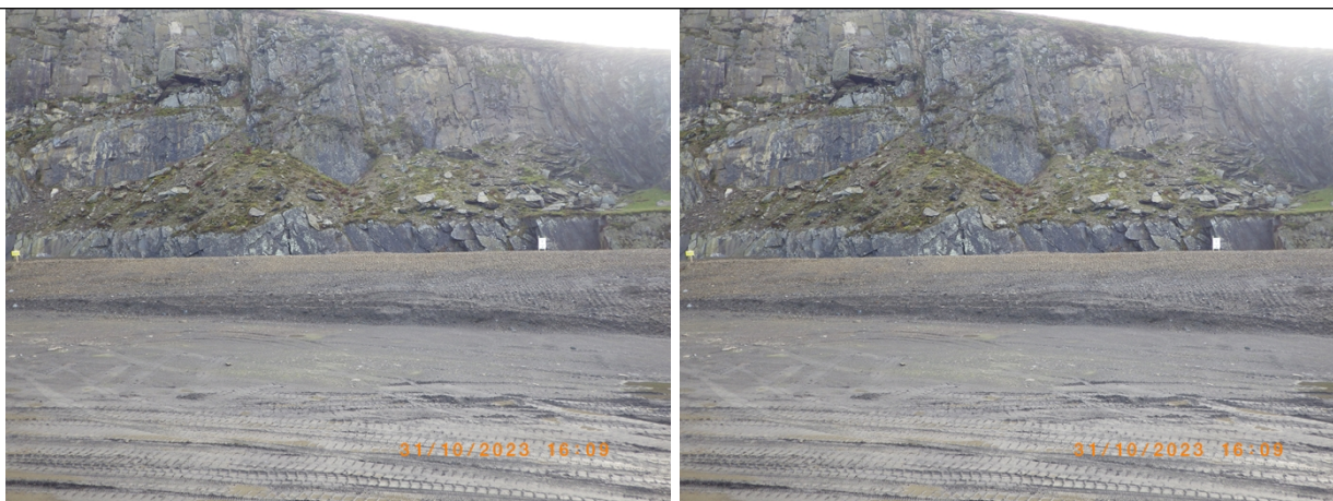
Lagoon area of the quarry filled with waste material
