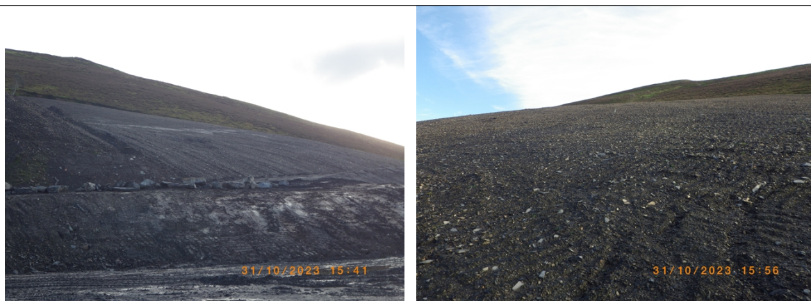
Levelled area of the quarry in preparation for remediation
