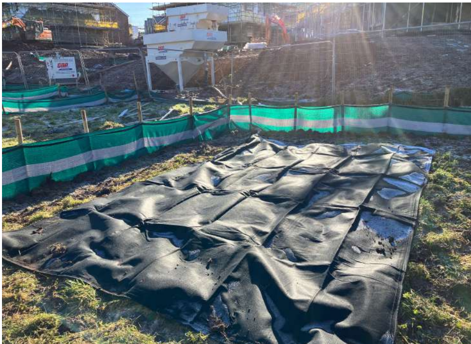
Photo 10 – Geobag final polishing treatment
