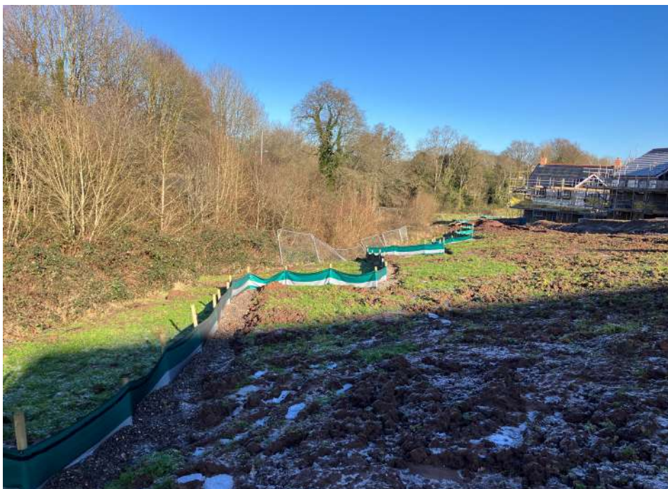
Photo 14 – Maintain Silt Fence along the perimeter to prevent runoff into stream
