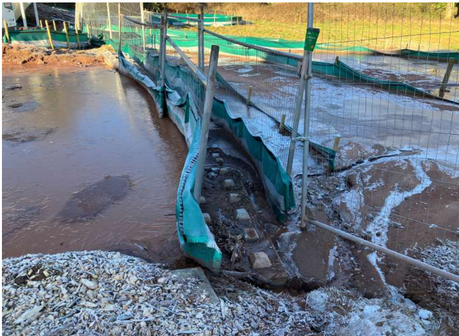
Photo 2 – Attenuation ponds have deep unconsolidated mud
