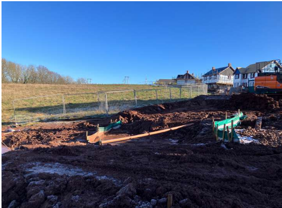
Photo 13 – Bund the site perimeter to direct water to settlement basins
