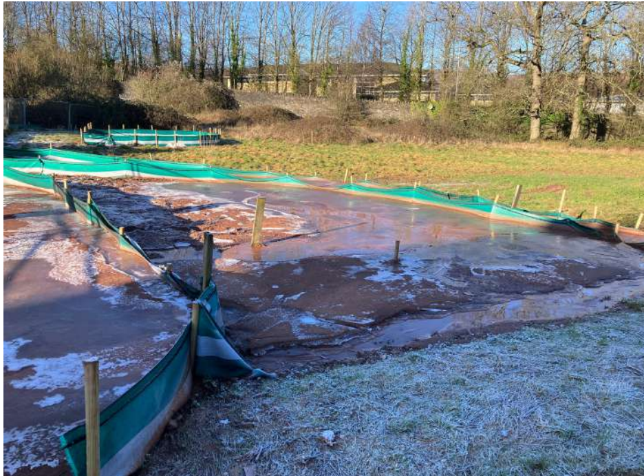
Photo 3 – Attenuation ponds have deep unconsolidated mud
