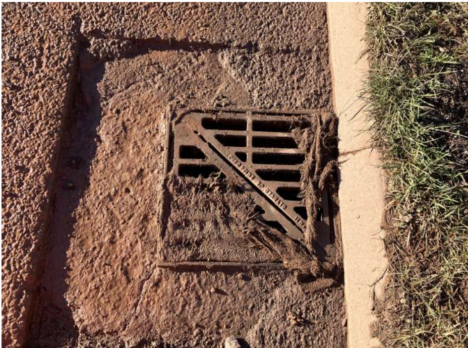
Photo 20 – Drainage covers require maintenance
