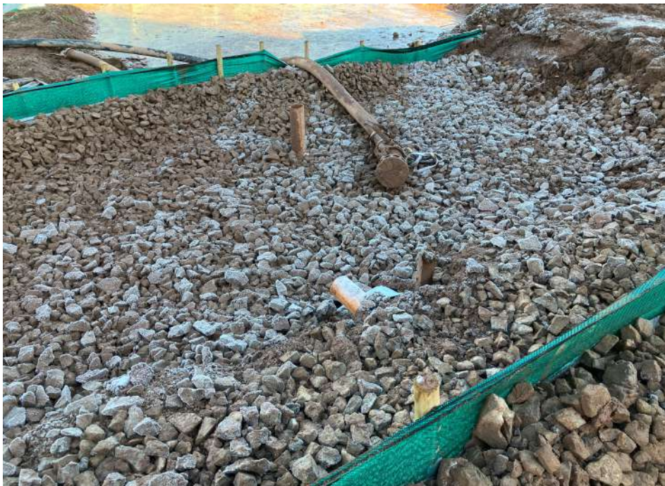
Photo 8 – Creation of new settlement pond on the site boundary
