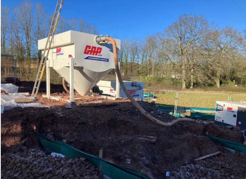
Photo 9 – Adapt settlement tank and confirm fit for purpose
