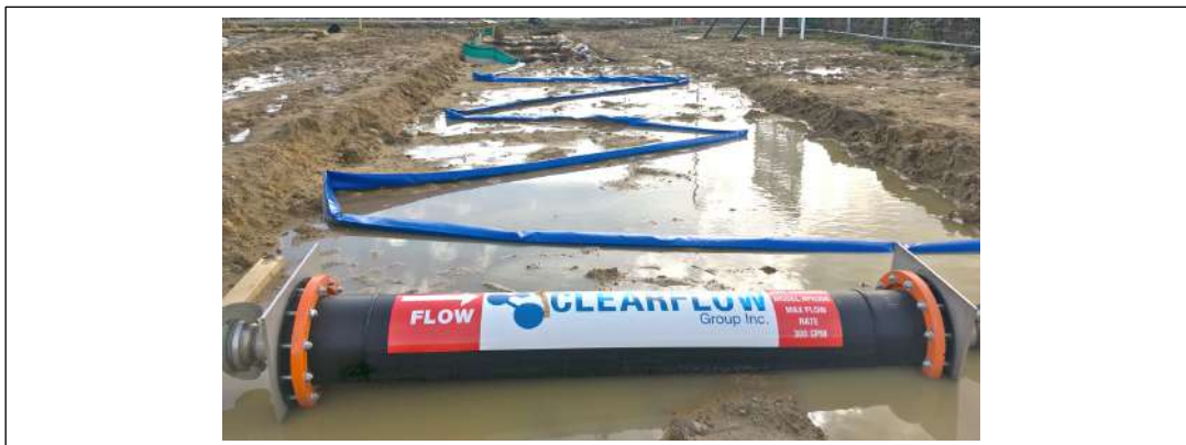
Photo 12 – The use of a Pipe Reactor to treat water pumped off site
