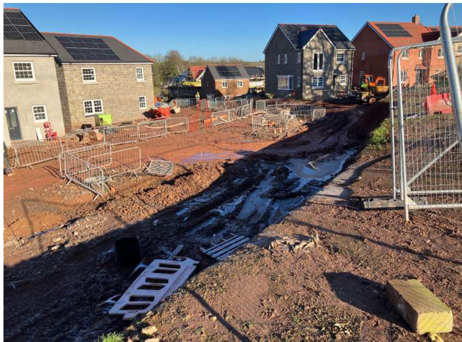
Photo 17 – Bund and divert water from top section of plot
