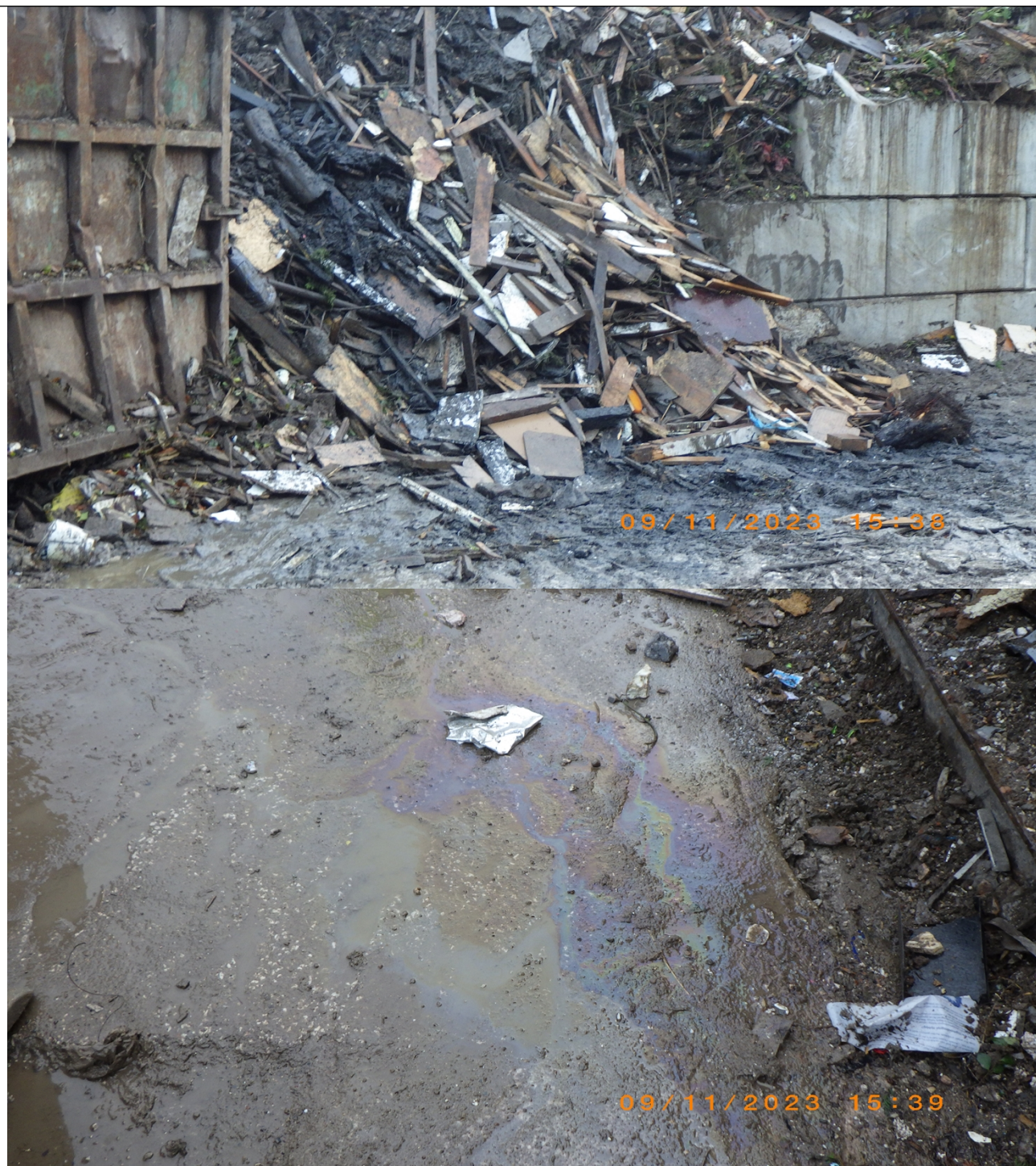
Photographs showing oil contamination on site
