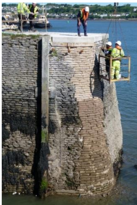
Photo 9 - Crane and basket to carry operatives for wall repairs
