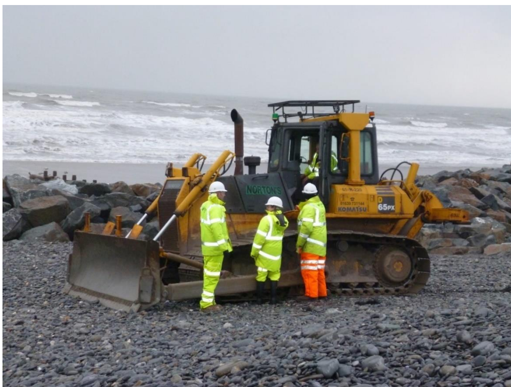
Photo 5 - Dozer to spread out the shingle
