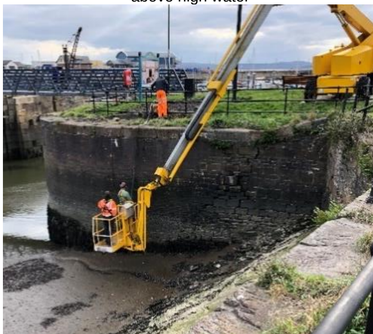
Photo 9 - Crane and basket to carry operatives for wall repairs
