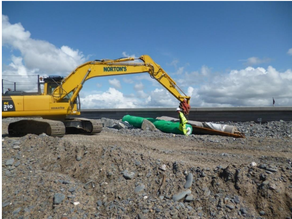
Photo 3 – Tracked excavator with a grab to pick up and place rock
