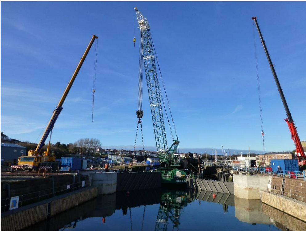
Photo 12 – Barge, Crane and Gate at Milford Marina
