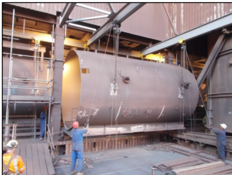
Figure 1 - North Windmain Replacement
