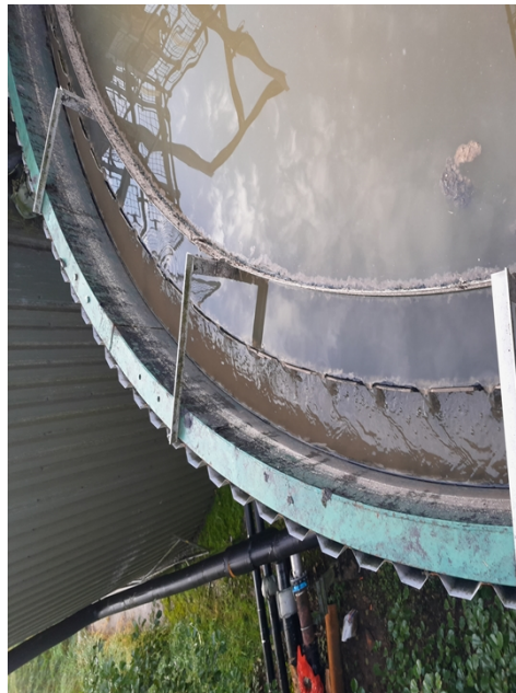
Solids carried into outlet channels from PSTs
