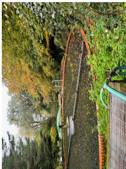
Filter beds - moss growth, leaf litter and ponding on filter medium.
