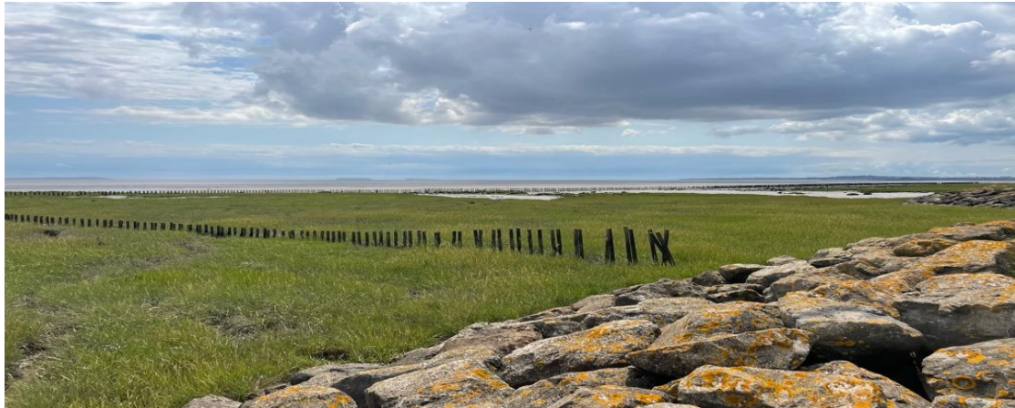
Above Rock Armor to remove and replace or ramp over at access points
