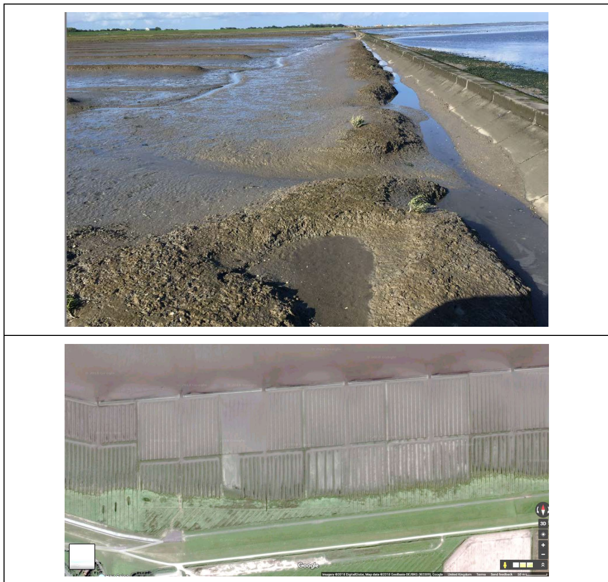
Figure 32. Images of a concrete seaward toe of the Polder system at the outer Querlahnung
