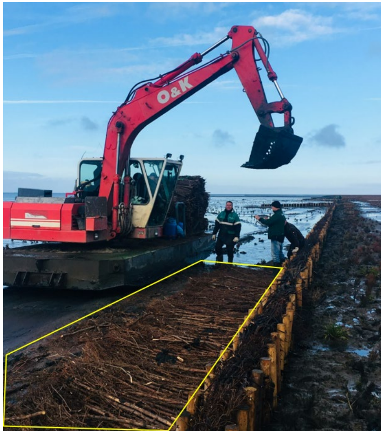
Figure 34. Example of scour protection using brushwood
