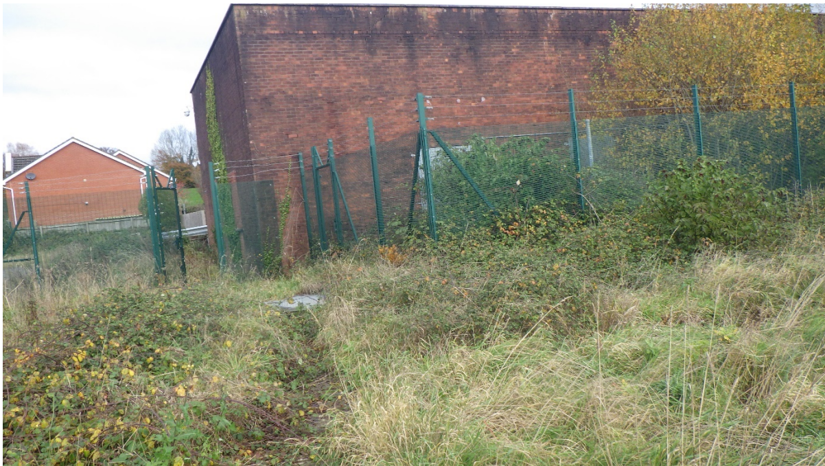
Figure 5: Site Visit Photos – access to storm tanks at the rear of the compound.
