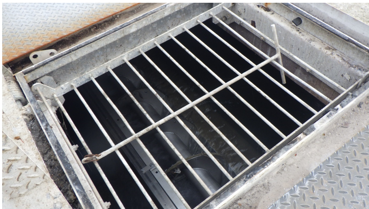
Figure 2: Site visit photo – high flow visible prior to effluent screening.
