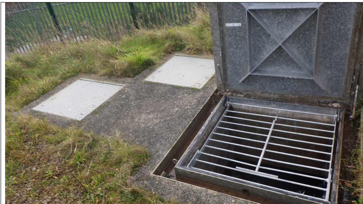
Figure 8: Site visit photo – Final inspection/access point before storm line leaves site.
