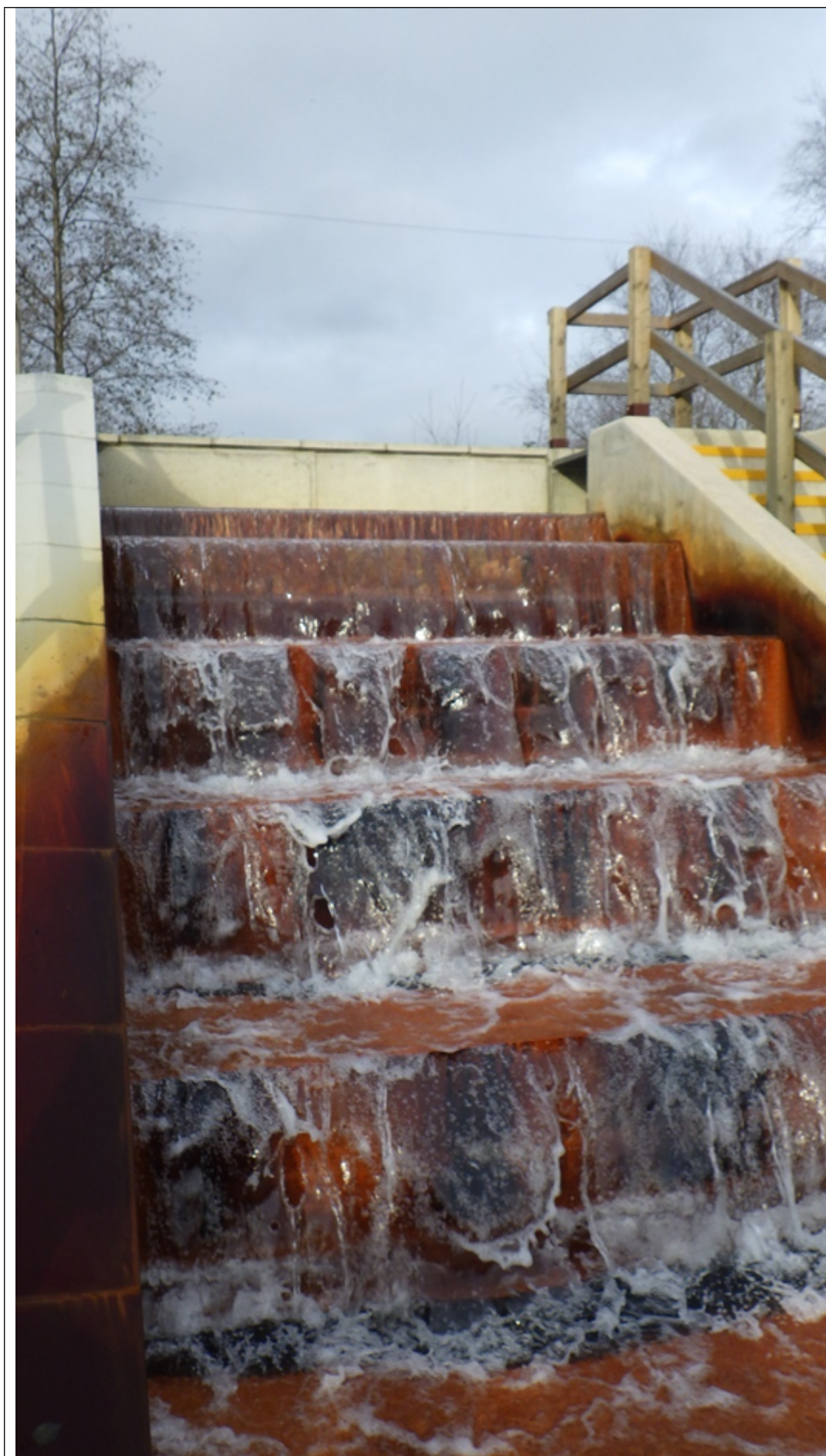
Figure 1 – Site visit photo: The condition of the cascade at the time of the visit. www.naturalresourceswales.gov.uk
