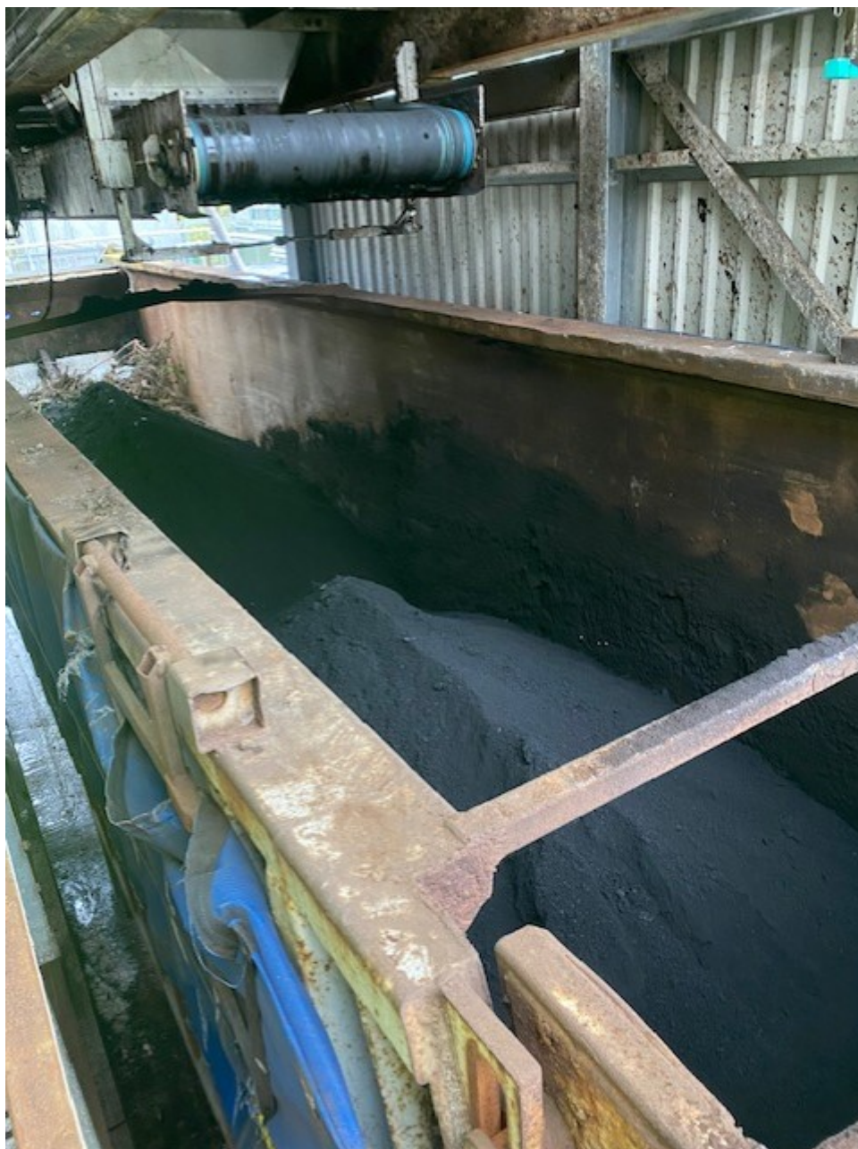
Photo 1. Hopper and Belt Discharge Point.
