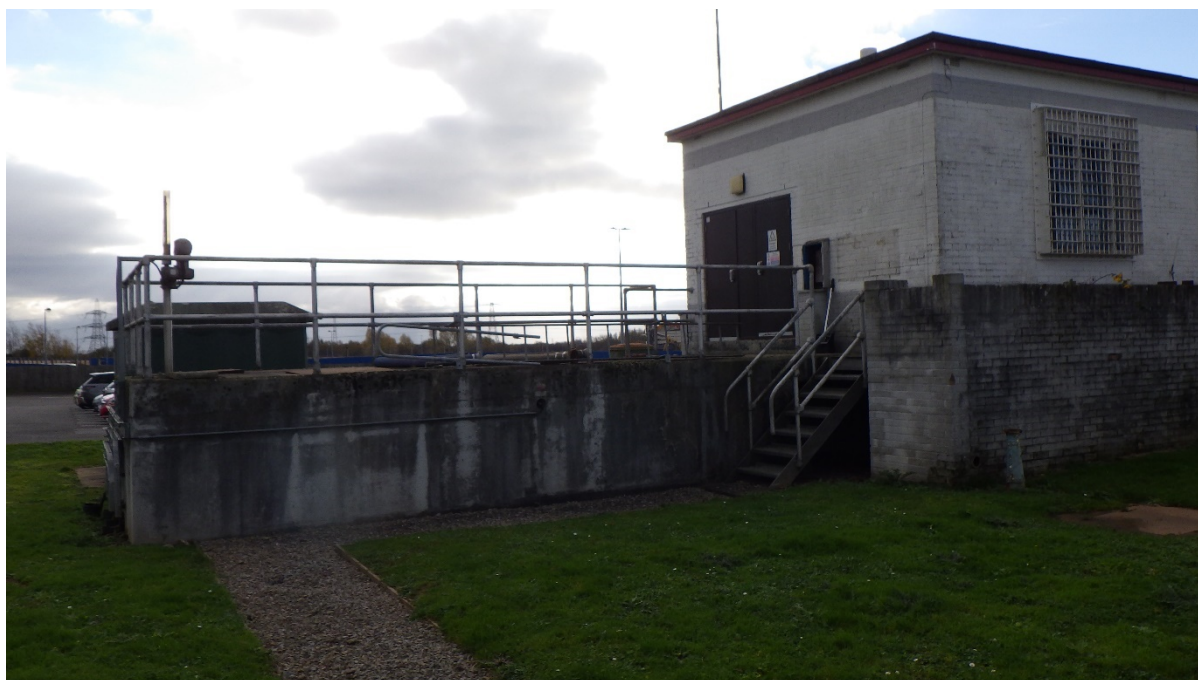
Figure 7: Site visit photo – Clearly accessible DCWW asset where the sample point is located.
