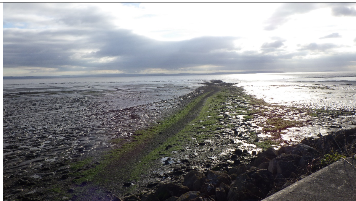
Figure 9: Site visit photo – Storm outfall submerged and inaccessible at the time of the visit.
