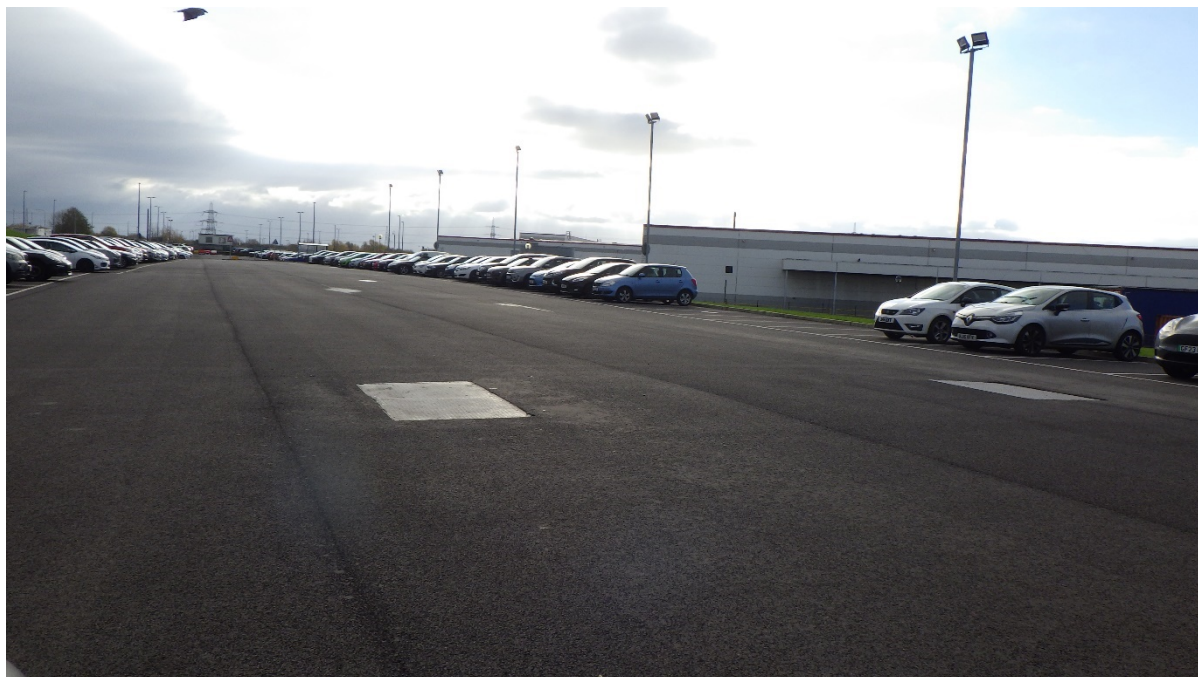
Figure 6: Site visit photo – Access points to storm tanks clear of obstructions.
