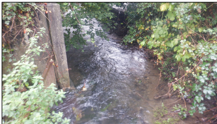
Image 5 - showing the Afon Arad below the penstock sluice gate running clear, taken at 12:05 on 19 October 2023
