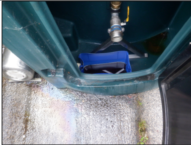
Image 6 (b) – showing oil storage hatch opening and sheen to the left of vessel, taken at 11:15 on 19 October 2023
