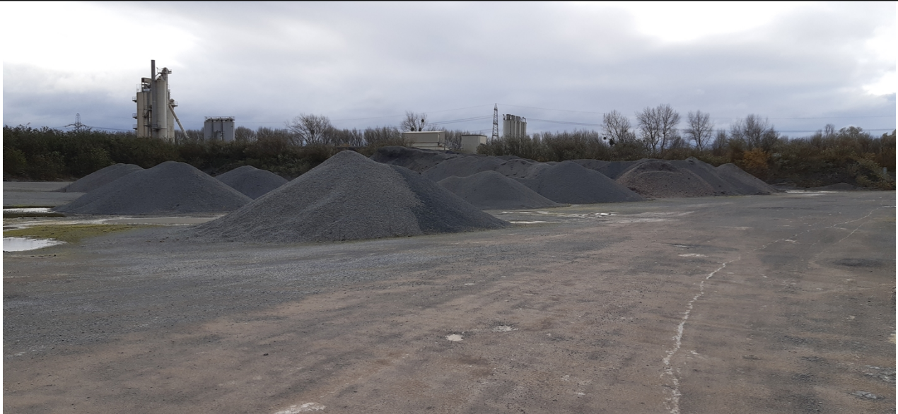
Photo 1 - Stockyard area of Tarmac Trading Ltd, Llanwern
