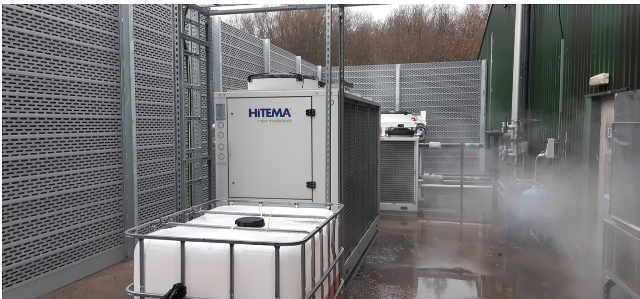
Photo 4 - Recently installed noise barrier to mitigate excess noise
