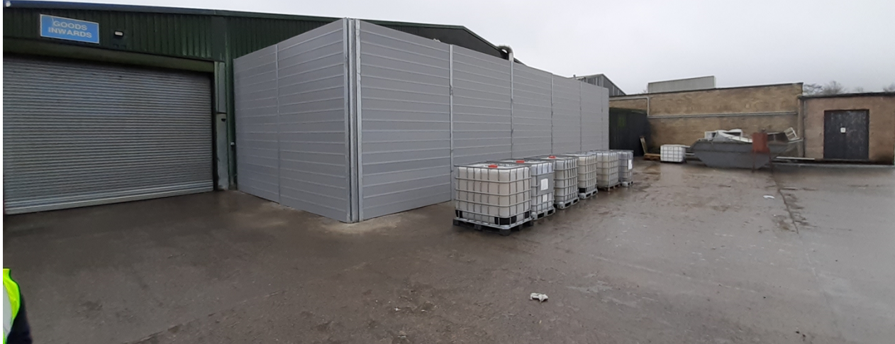
Photo 3 - Recently installed noise barrier to mitigate excess noise
