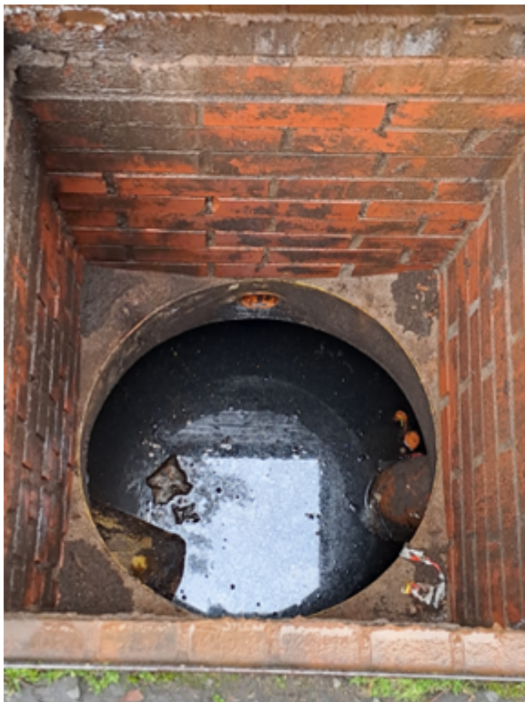
Figure 2. Contents of the primary interceptor chamber.
