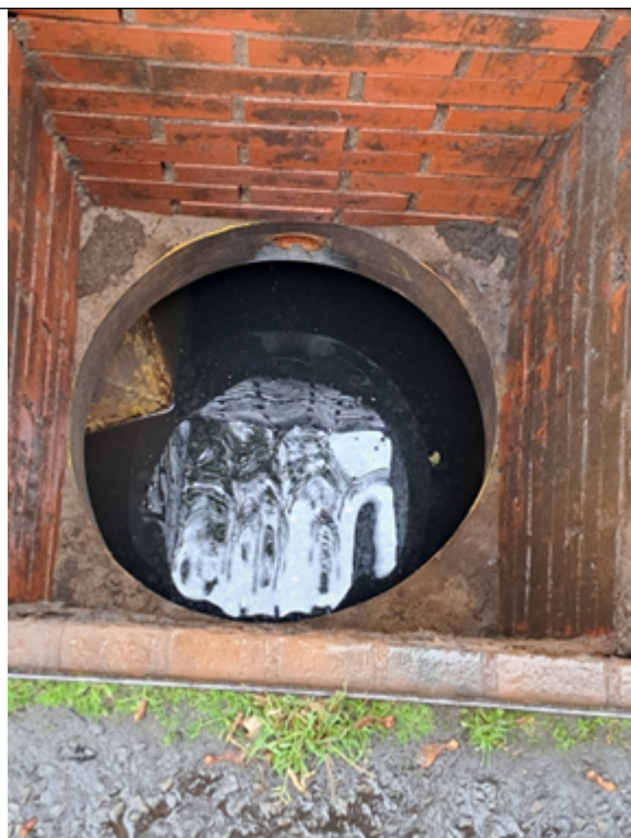
Figure 3. Contents of the secondary interceptor chamber.
