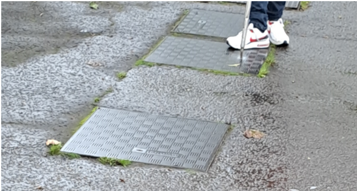
Figure 1. Location of the three interceptor chambers.
