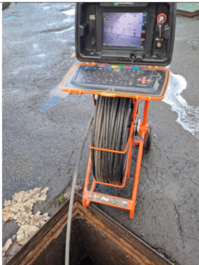
Figure 10. Evidence that the interceptor was connected to the soakaway system.
