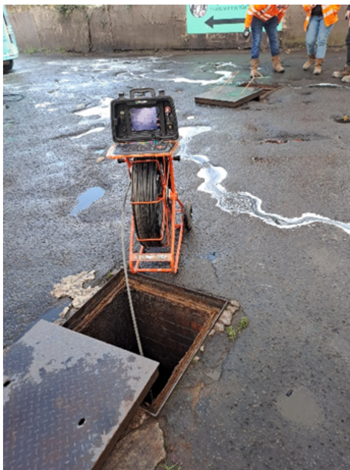
Figure 5. Location of the oil interceptor outlet/ soakaway inlet in the foreground, with the manhole over the soakaway in the background.
