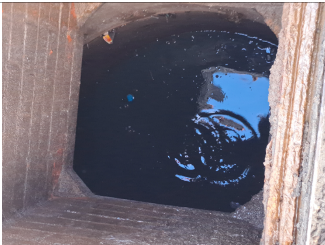
Figure 7. Contents of the soakaway system where oil and detergent can be observed.
