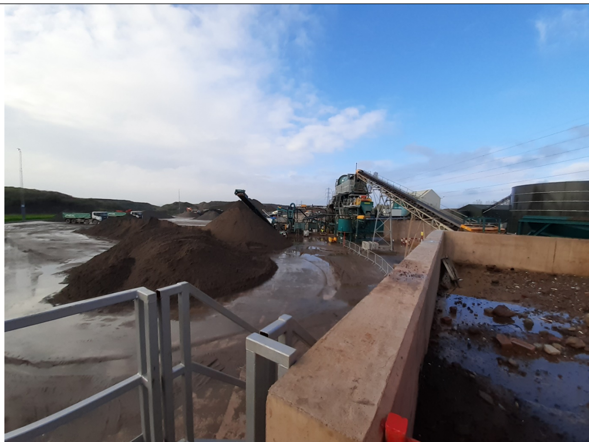
Figure 3 - Overall view of the wash plant and the material being deposited from the plant
