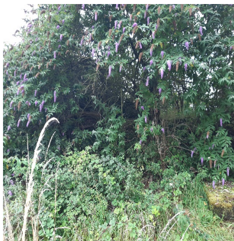
Figure 4: Discharge point inaccessible due to overgrowth
