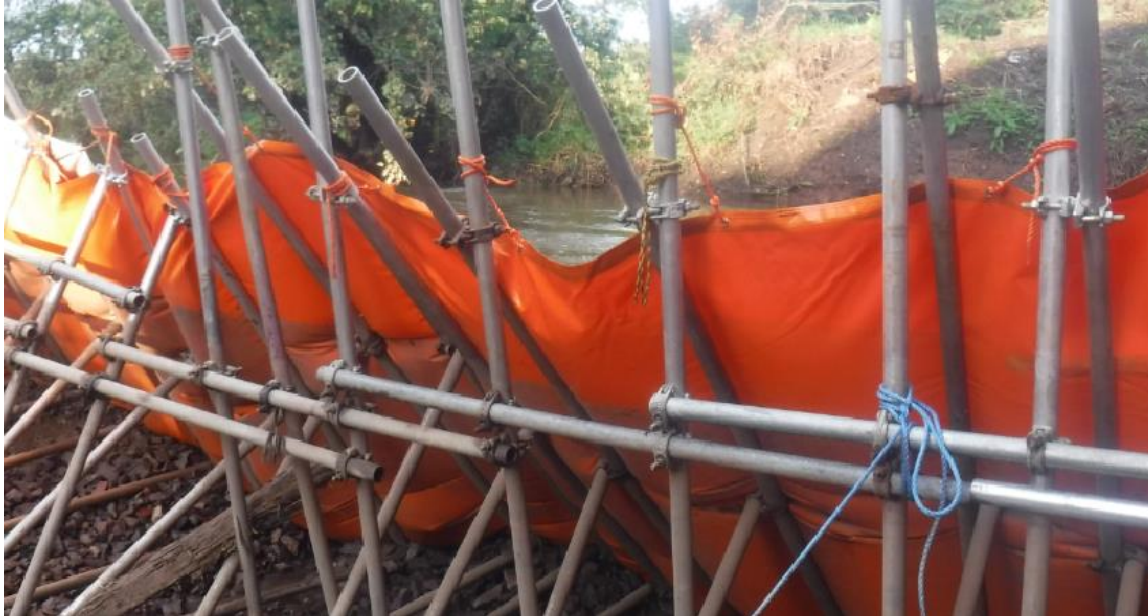
Figure 9: – Image highlighting the general frame dam arrangement.
