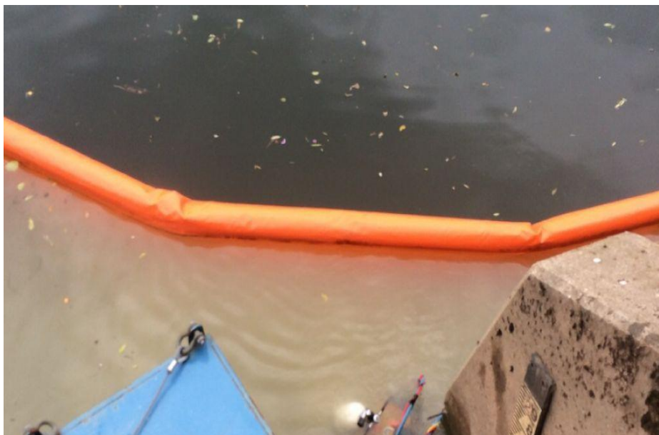
Figure 6: – Image highlighting a silt curtain capturing silt and fines.
