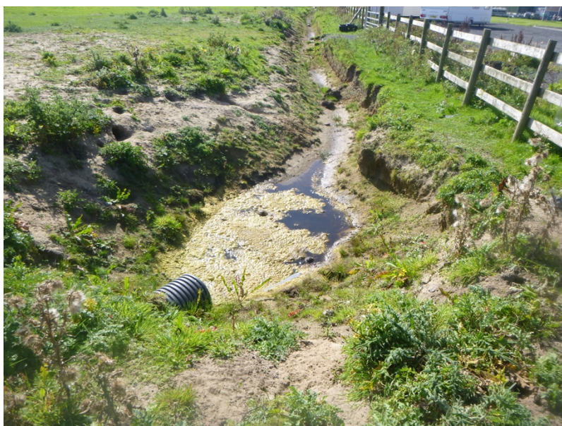
Photograph 4: Recently dug ditch potentially discharging into final effluent sample point
