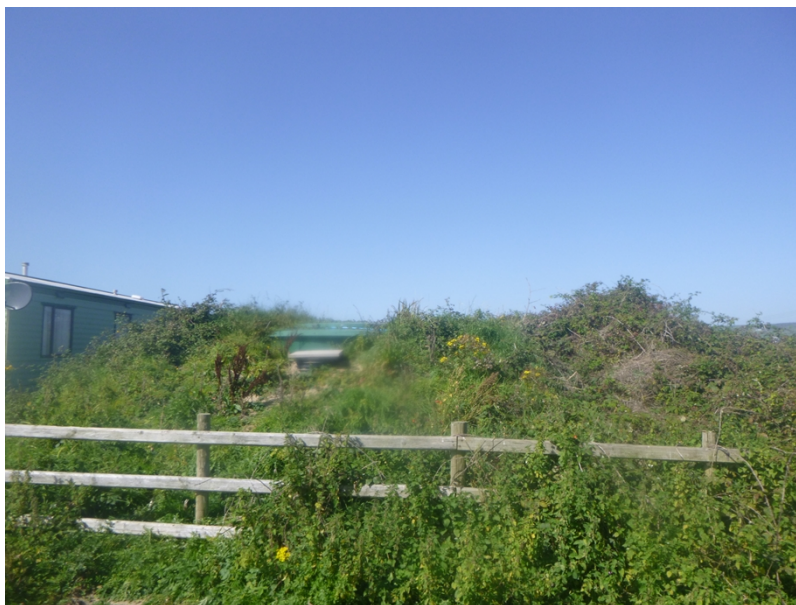
Photograph 1: Sewage Treatment Plant (STP) as viewed from ground level
