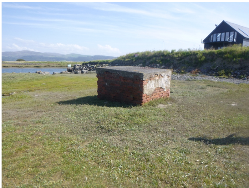
Photograph 6: Raised brick chamber
