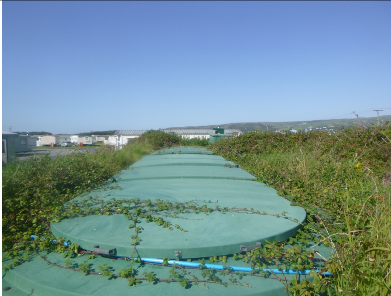
Photograph 2: Sewage Treatment Plant (STP) as viewed from above
