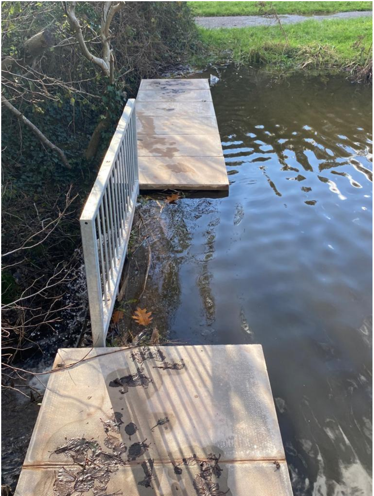
Repaired dam coping stones and barrier
