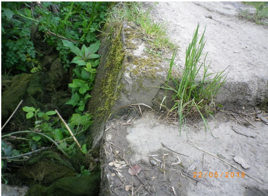
Degree of settlement to slab
