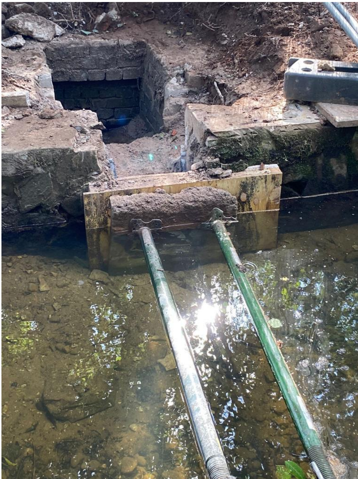
Uncharted manhole exposed during works
