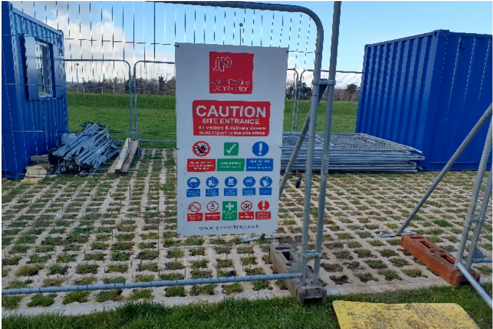
P4 Site safety signage displayed.
