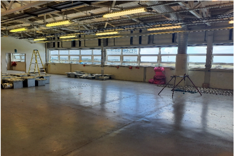
P2 Well managed work areas
