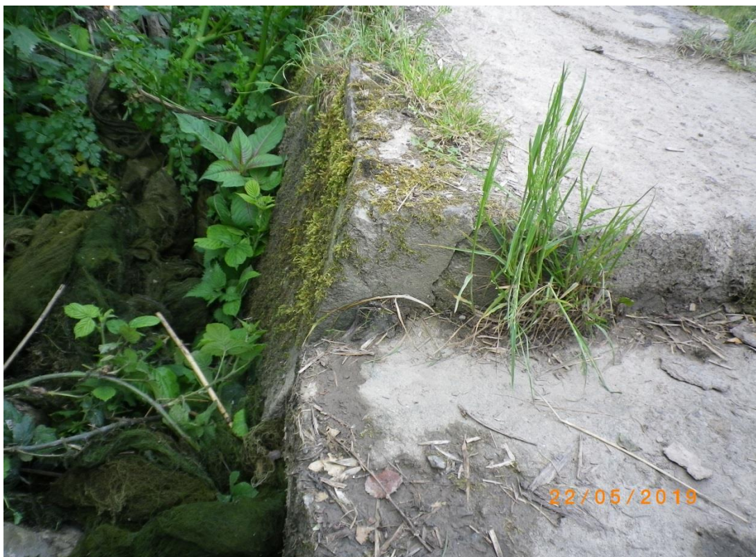
Degree of settlement to slab (PHOTO 4)
