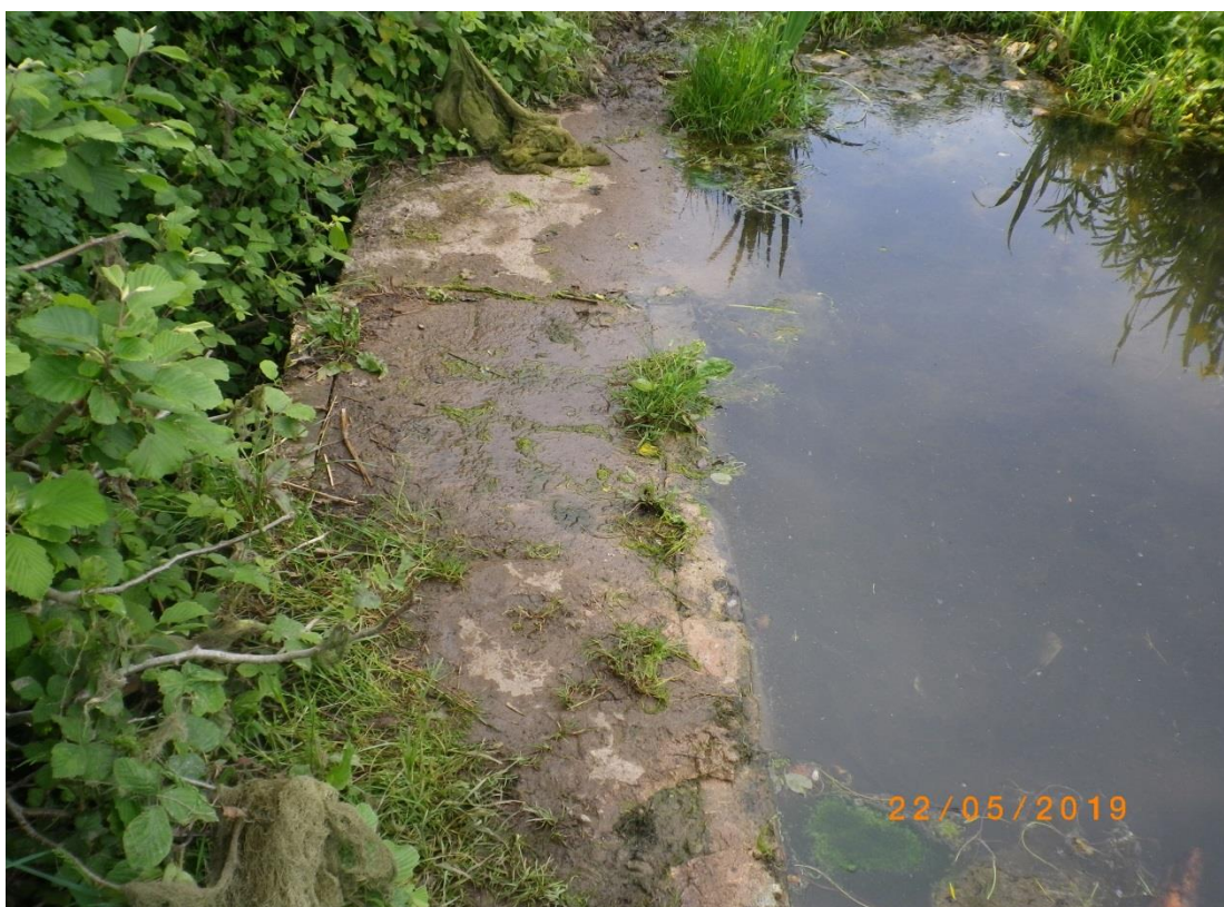
Overtopping of Dam wall (PHOTO 6)
