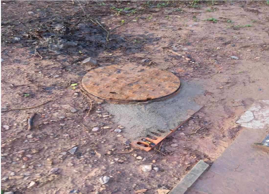
Previously uncharted manhole has been raised and exposed (PHOTO 14)
