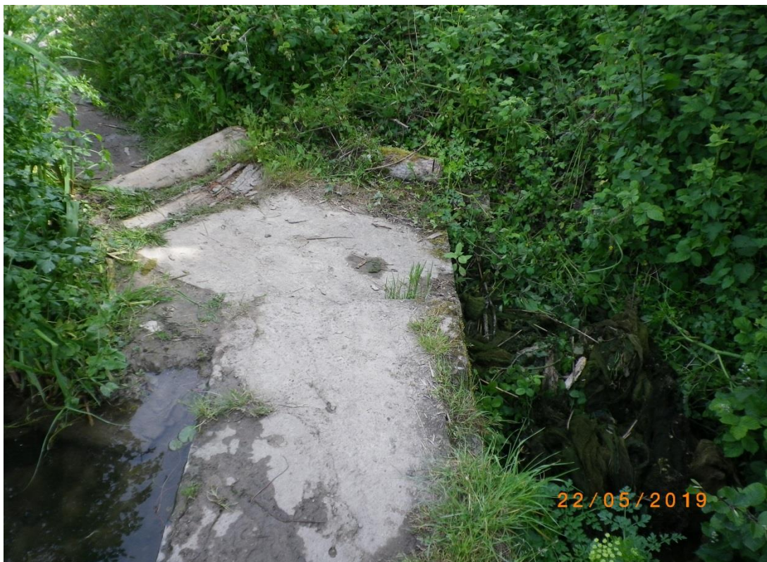
Sunken side slab (PHOTO 3)
