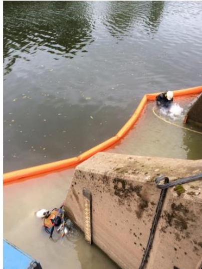
Figure 6: Example of how a Silt Curtain works.
