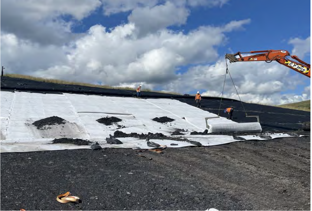
Overview of Work
