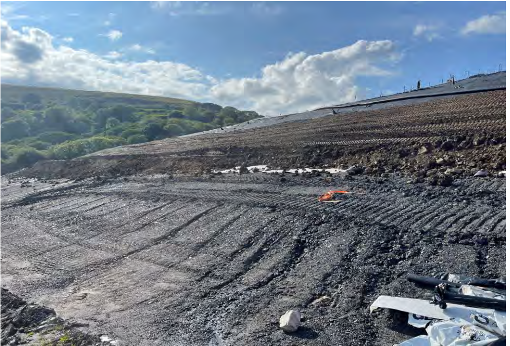
Overview of Work
