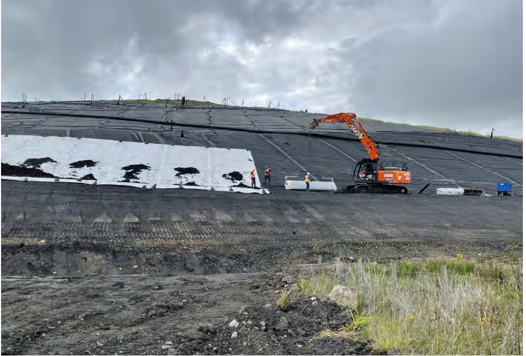
Continued GDL Installation
