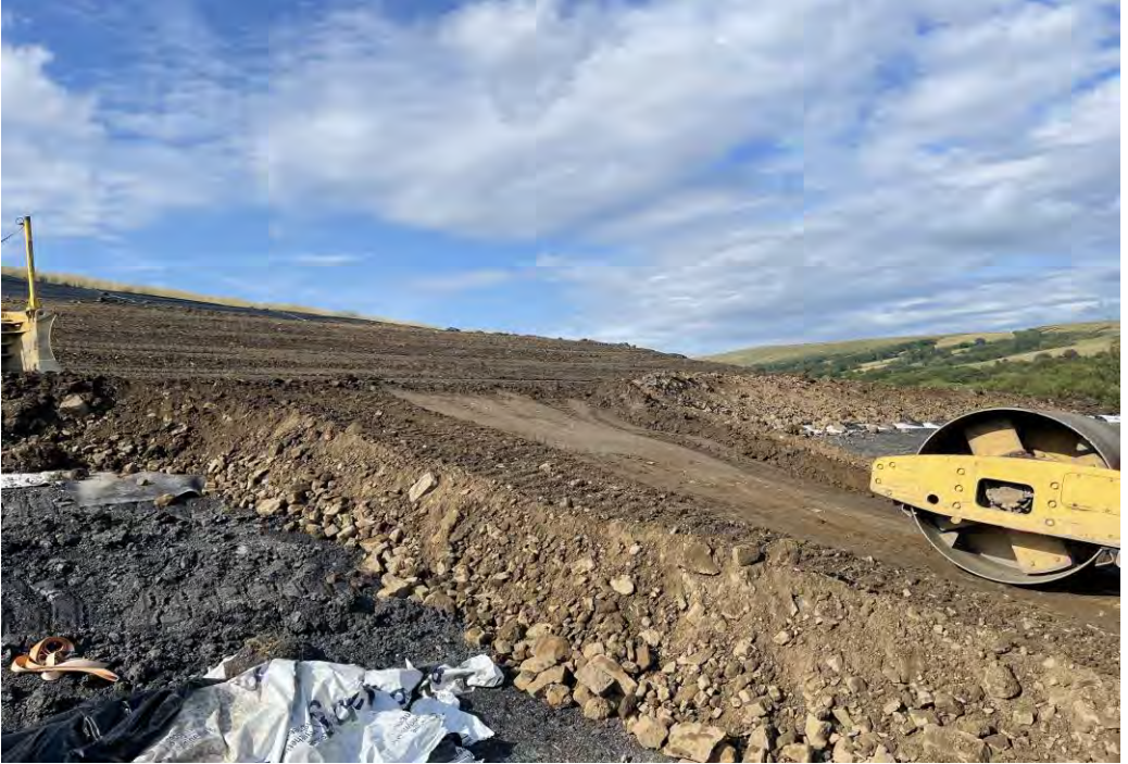
Restoration Placement in Progress
