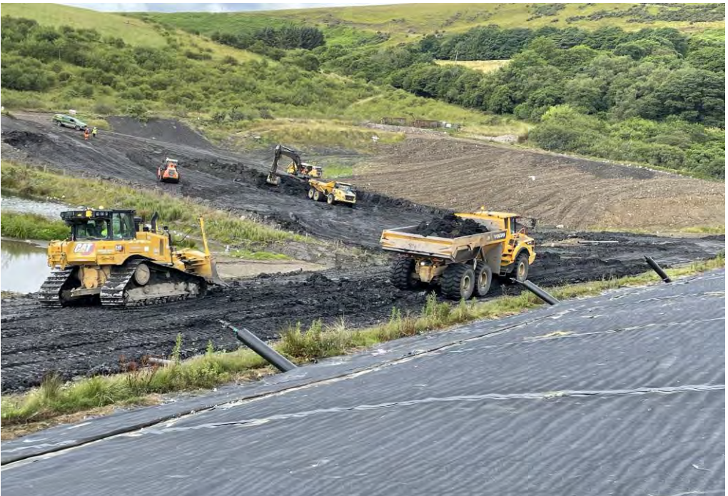
Preparing Working Area
