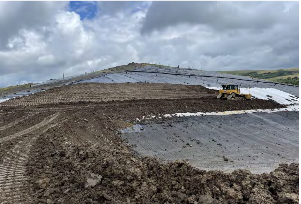
Restoration in Progress
