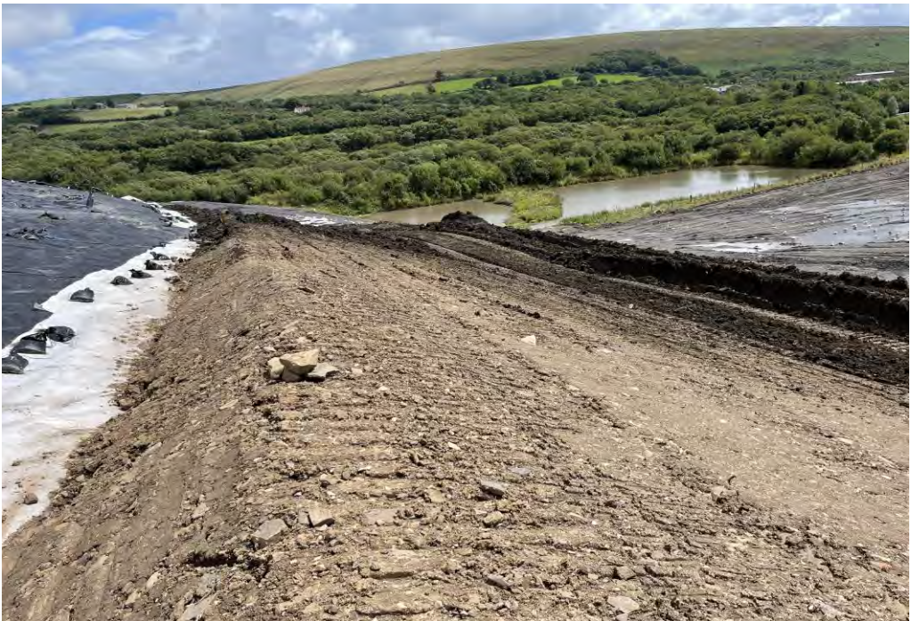
Overview of Work
