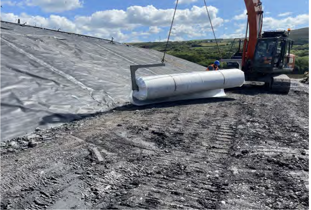
Preparing to Deploy GDL
