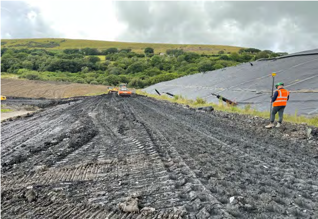
Compaction in Progress
