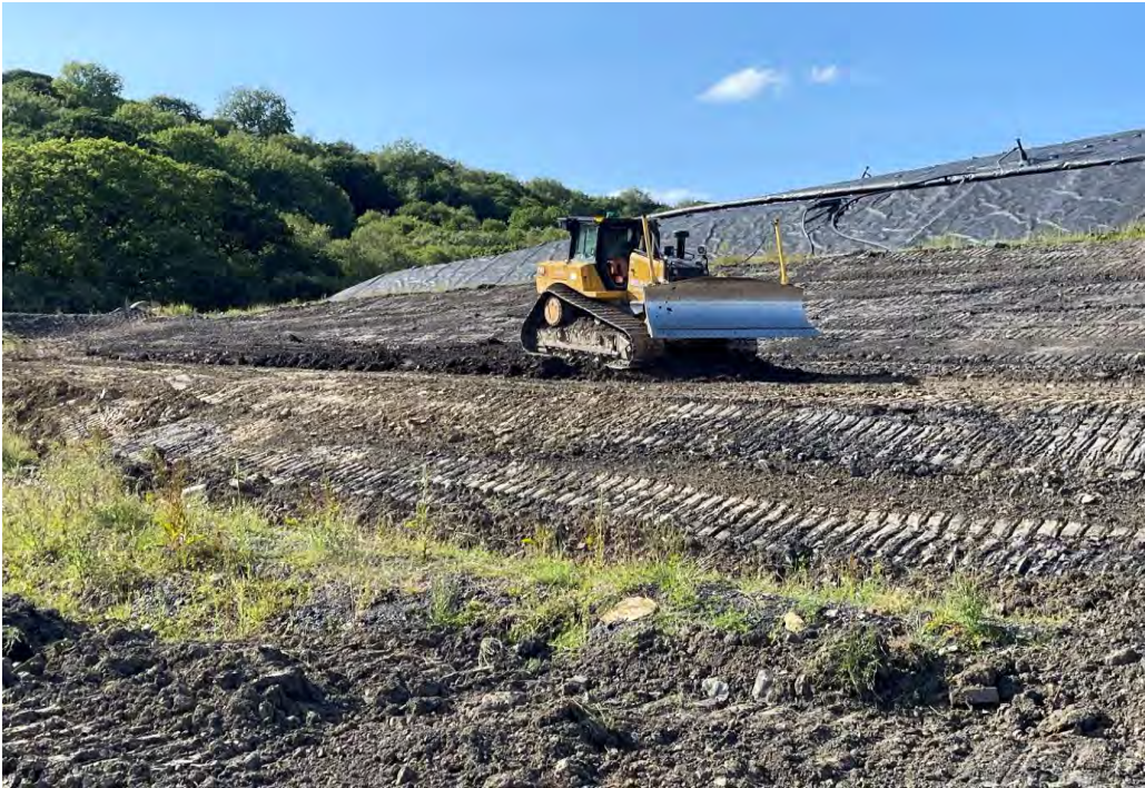
Continue to Install Buttress
