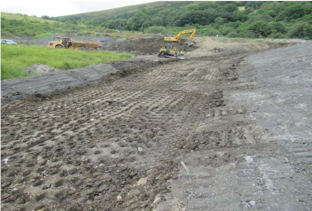
Compacted Buttress Material
