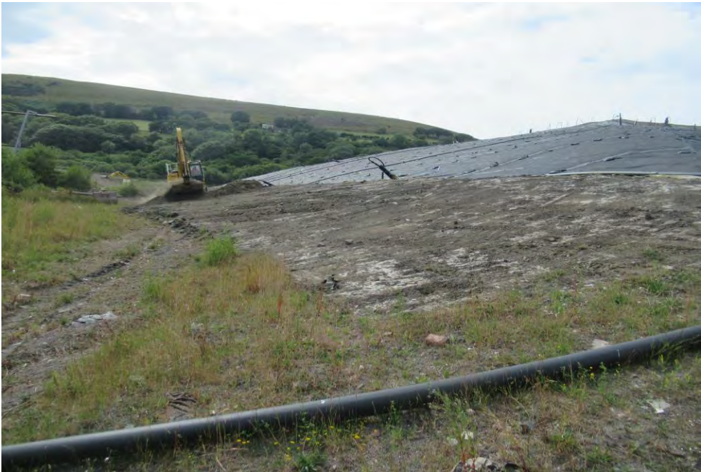
Clearing Vegetation For Buttress Works
