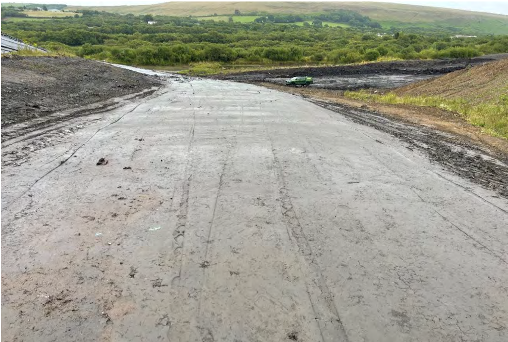
Overview of the Works
