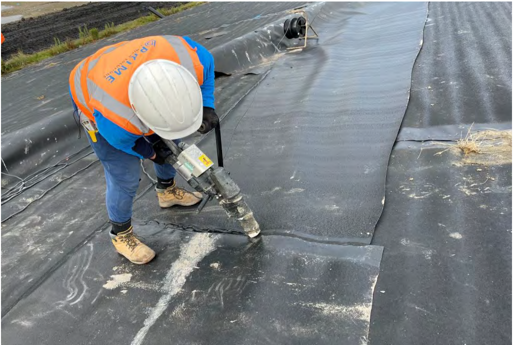
Extrusion Welding Diverted Rain Flap
