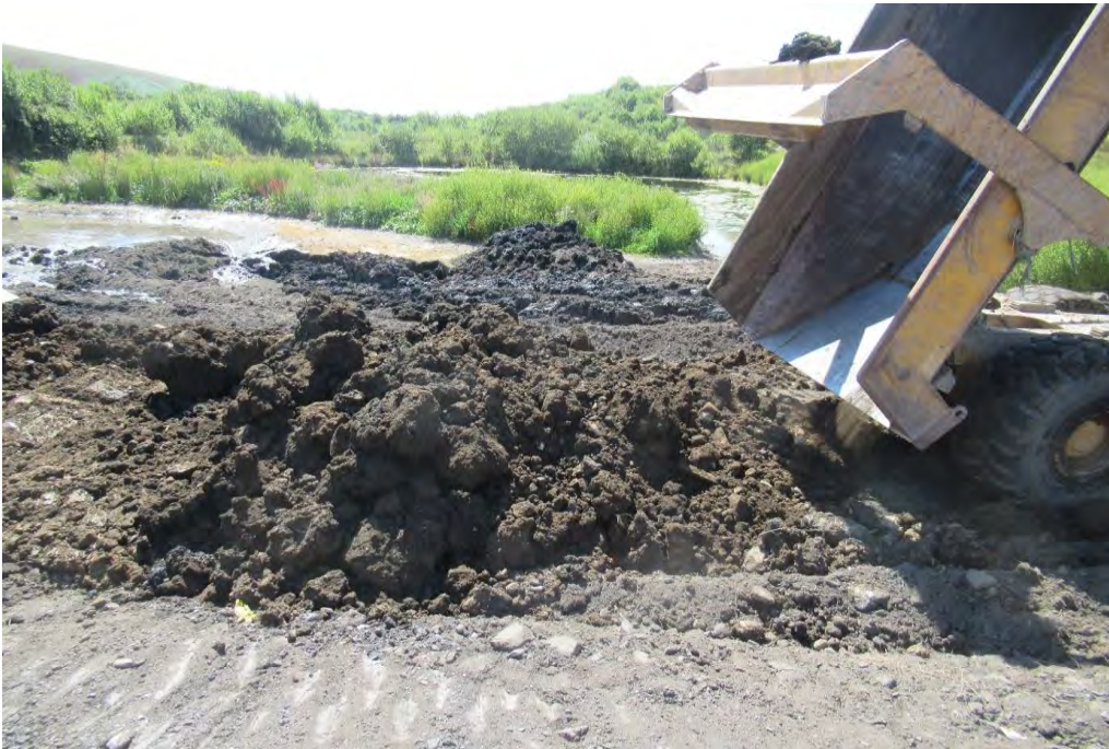
Tipping Off Of Buttress Material
