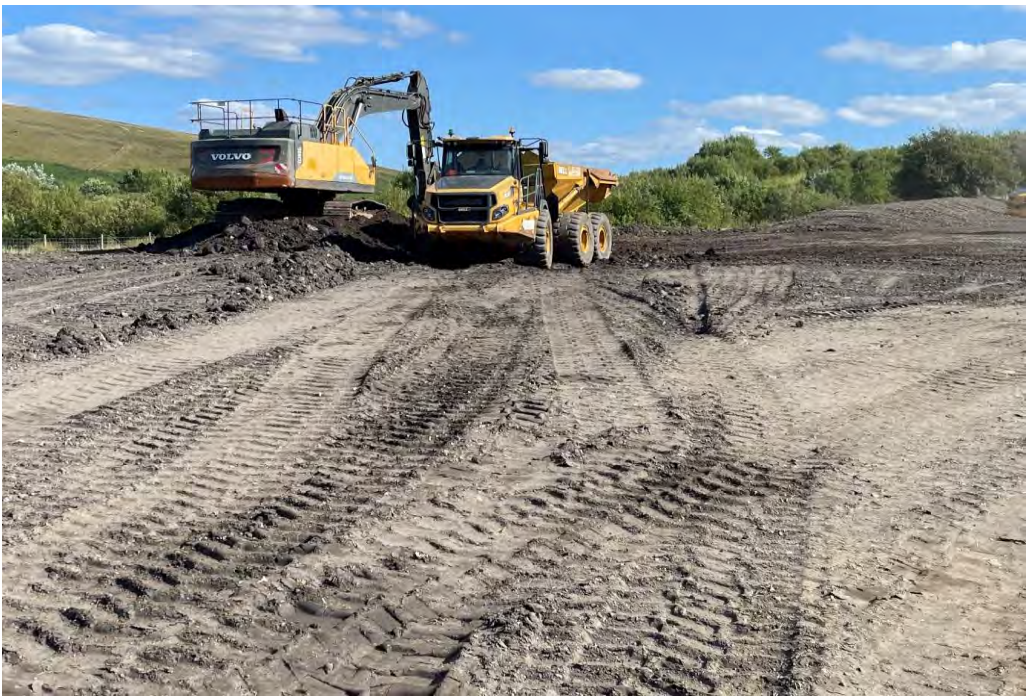
Loading Buttress Material
