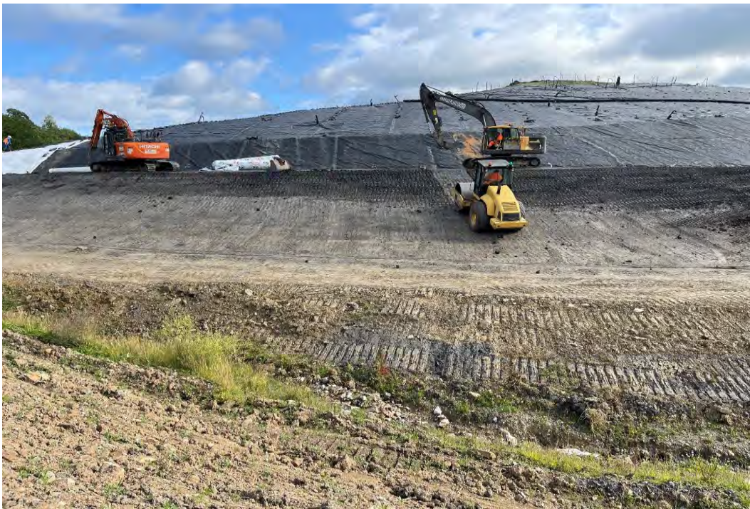
Smooth Drum Rolling Completed Buttress
