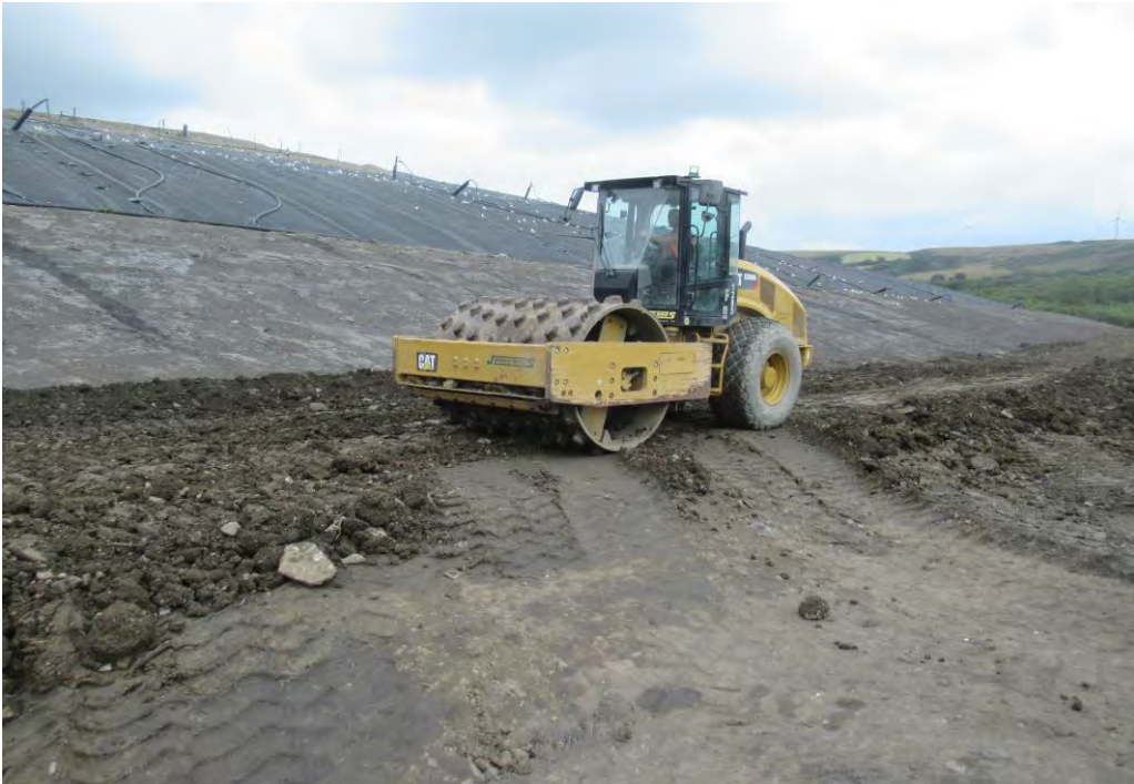
Compaction Of Buttress Material
