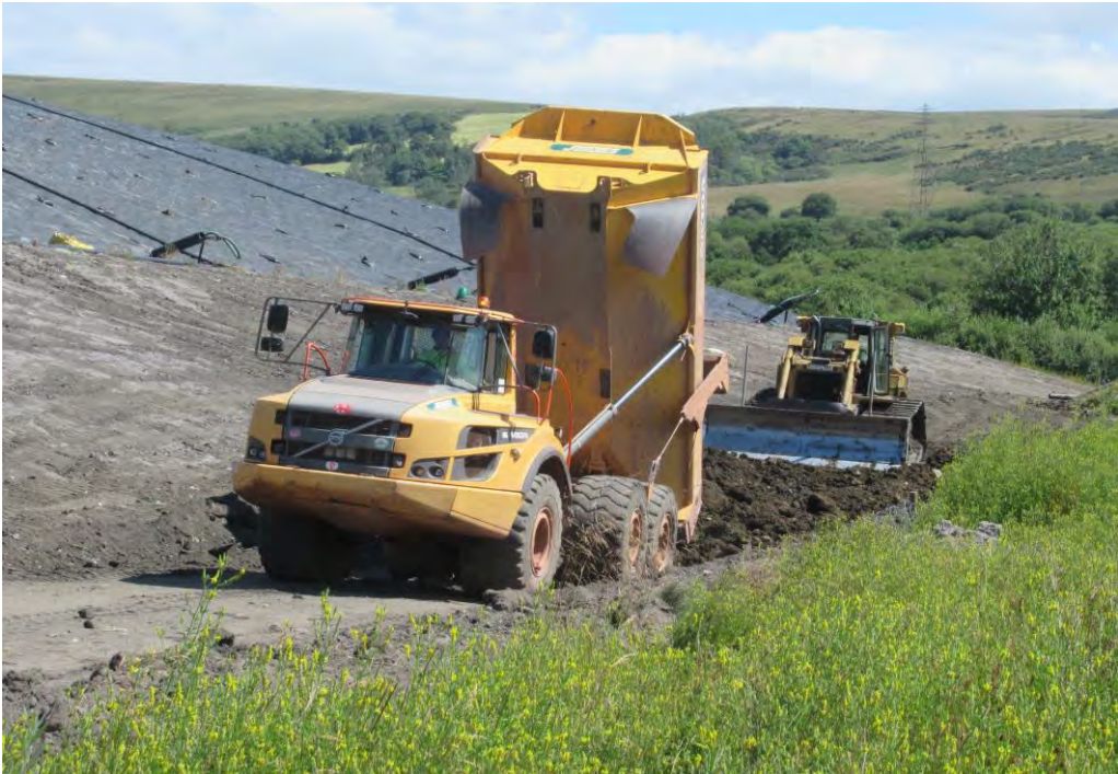
Placing Buttress Material
