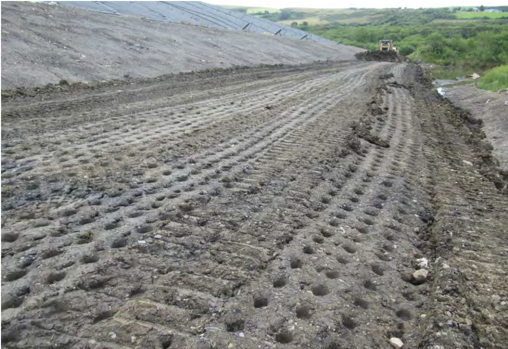
Compacted Material And Continued Placement Of Material
