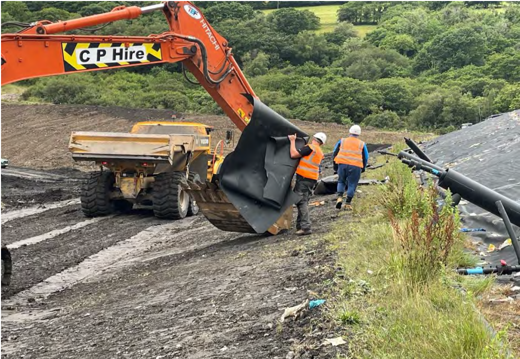
Loading Away Cut Out Rain Flap
