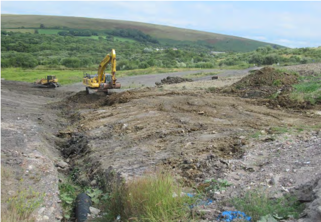
Buttress Work Begins
