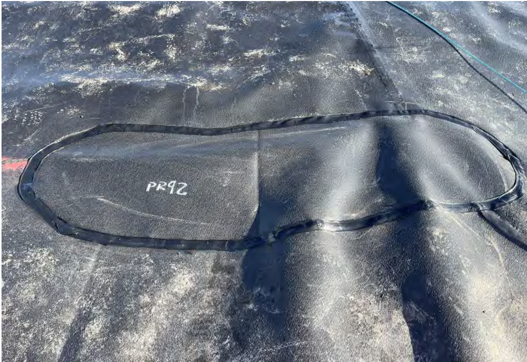
Completed Extrusion Welded Patch
