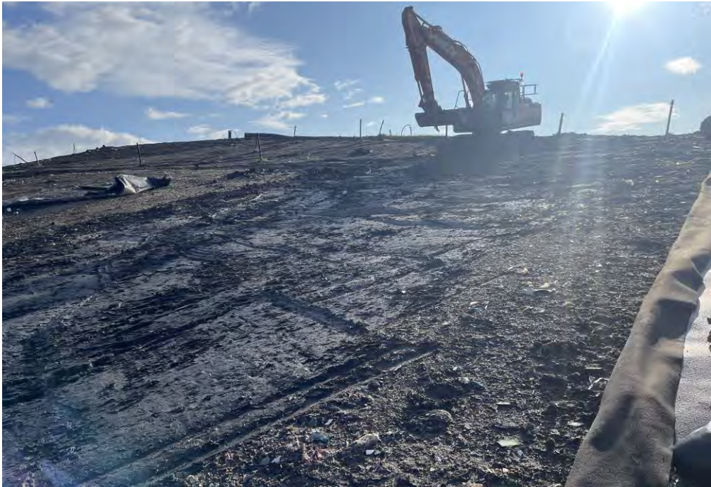
Regulating Layer Preparation
