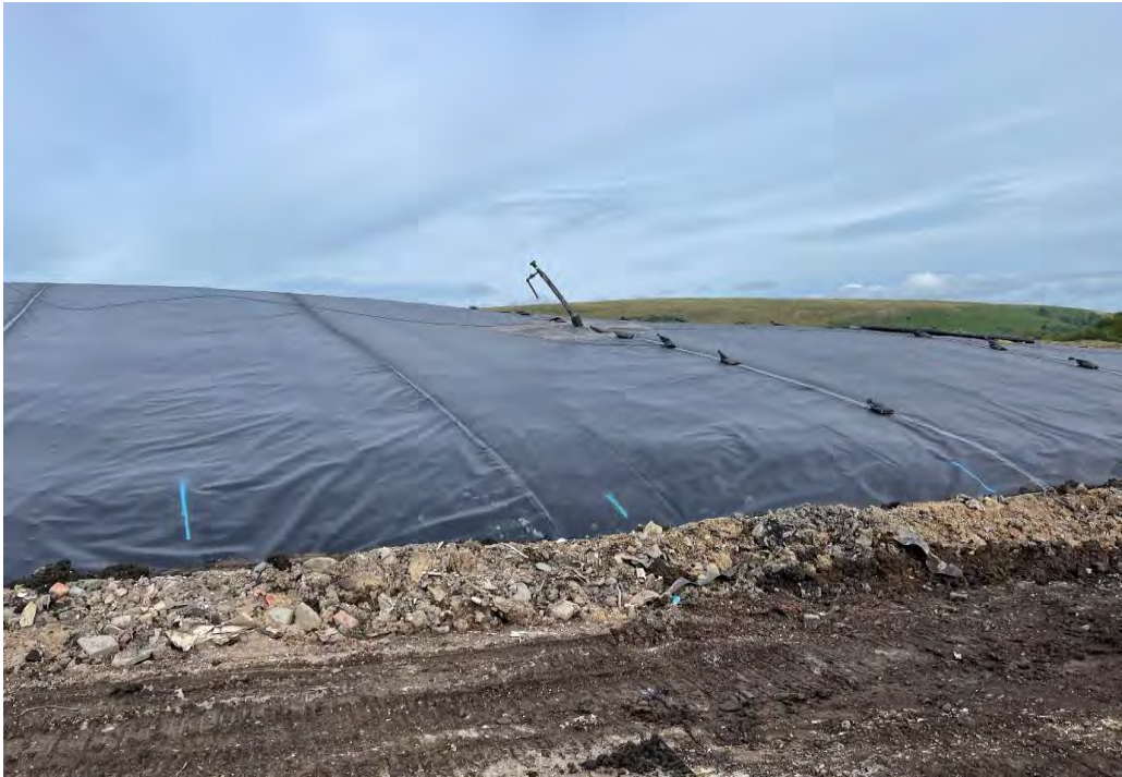
Completed Section of Capping
