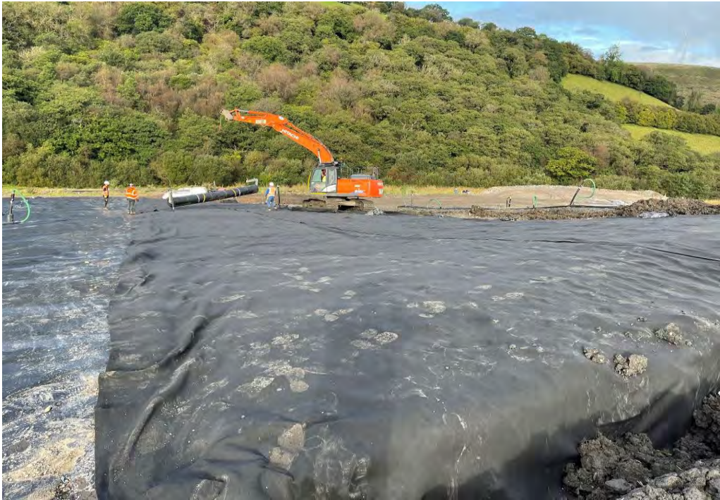
Installed Lower Geotextile
