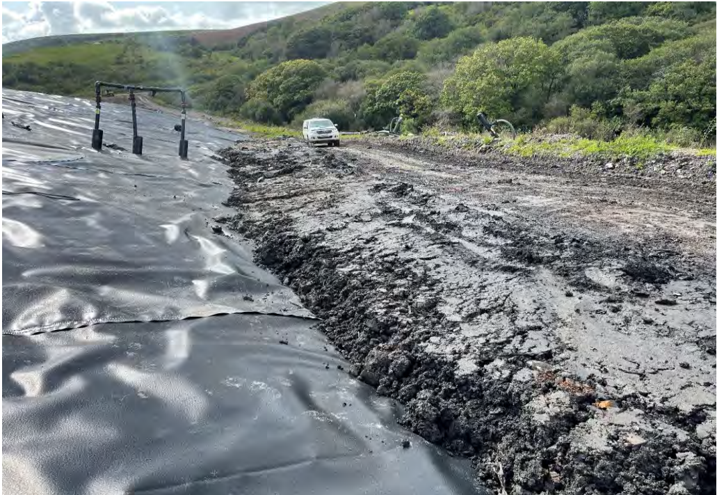
Completed Anchor Trench
