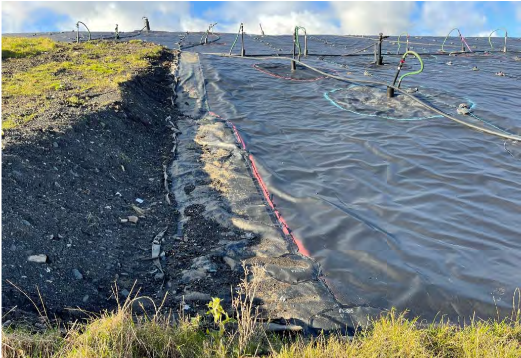
Completed Section of Tie in
