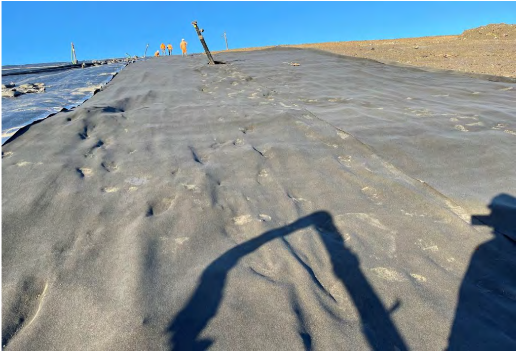
Installation of Lower Geotextile
