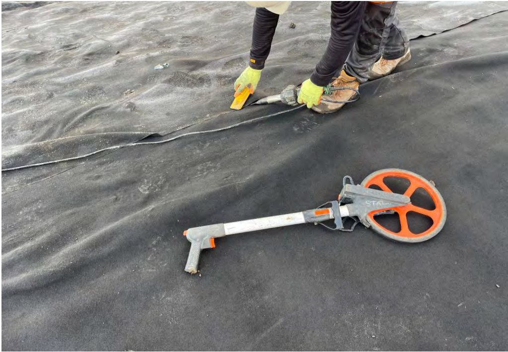
Heat Bonding Lower Geotextile
