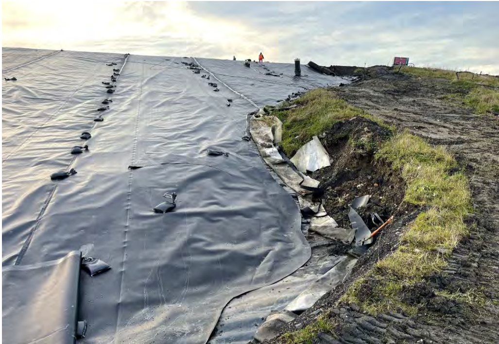
Geomembrane Installation Complete
