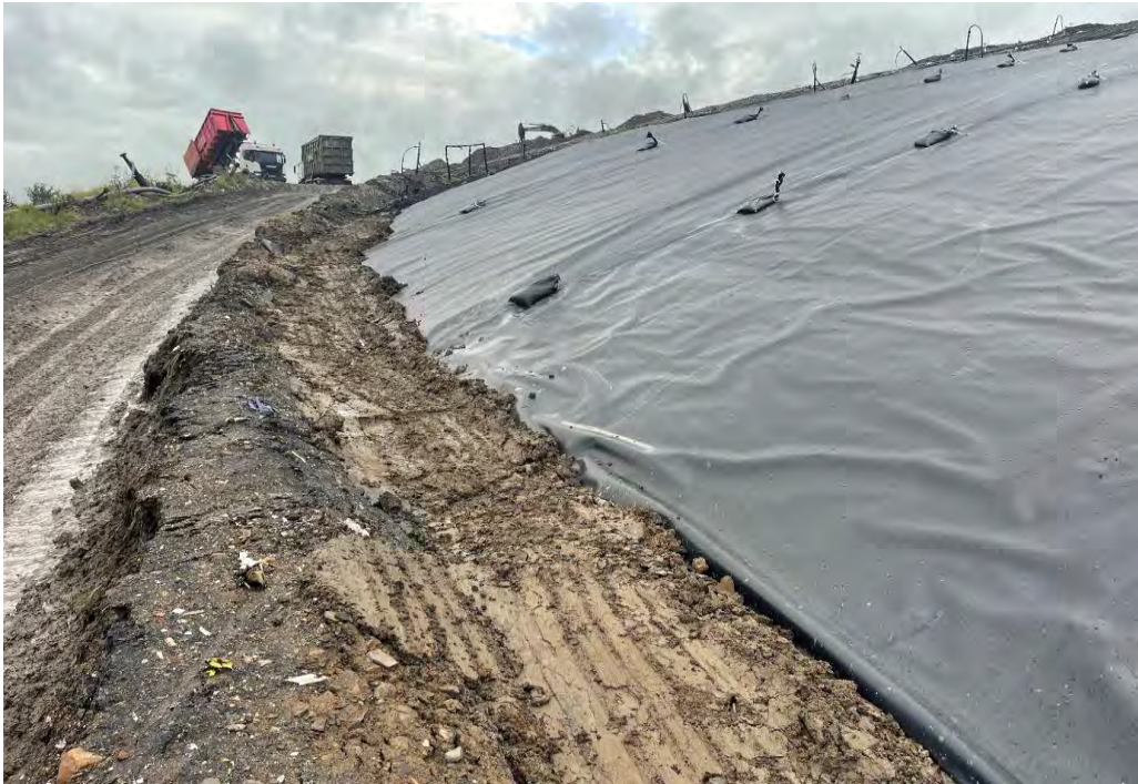
Completed Anchor Trench
