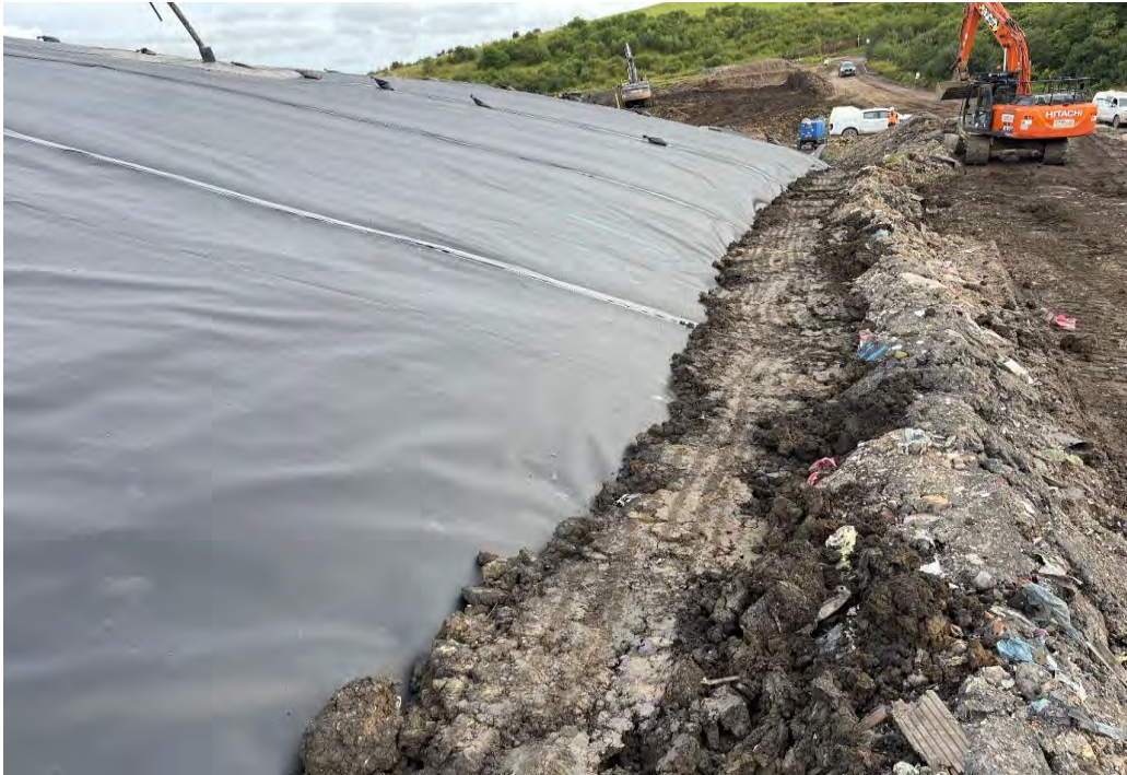
Completed Anchor Trench
