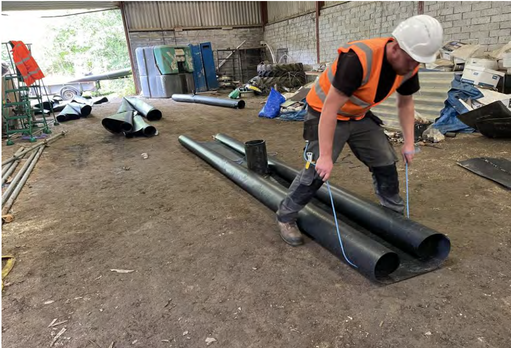
Prefabricating Pipe Boots
