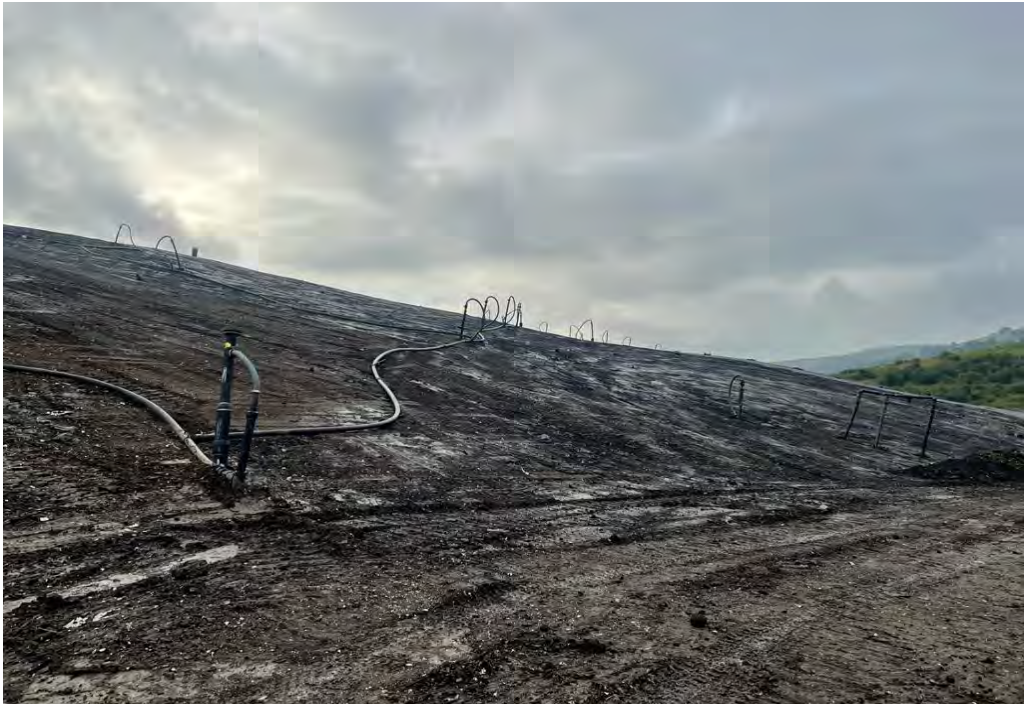
Ready for Lining
