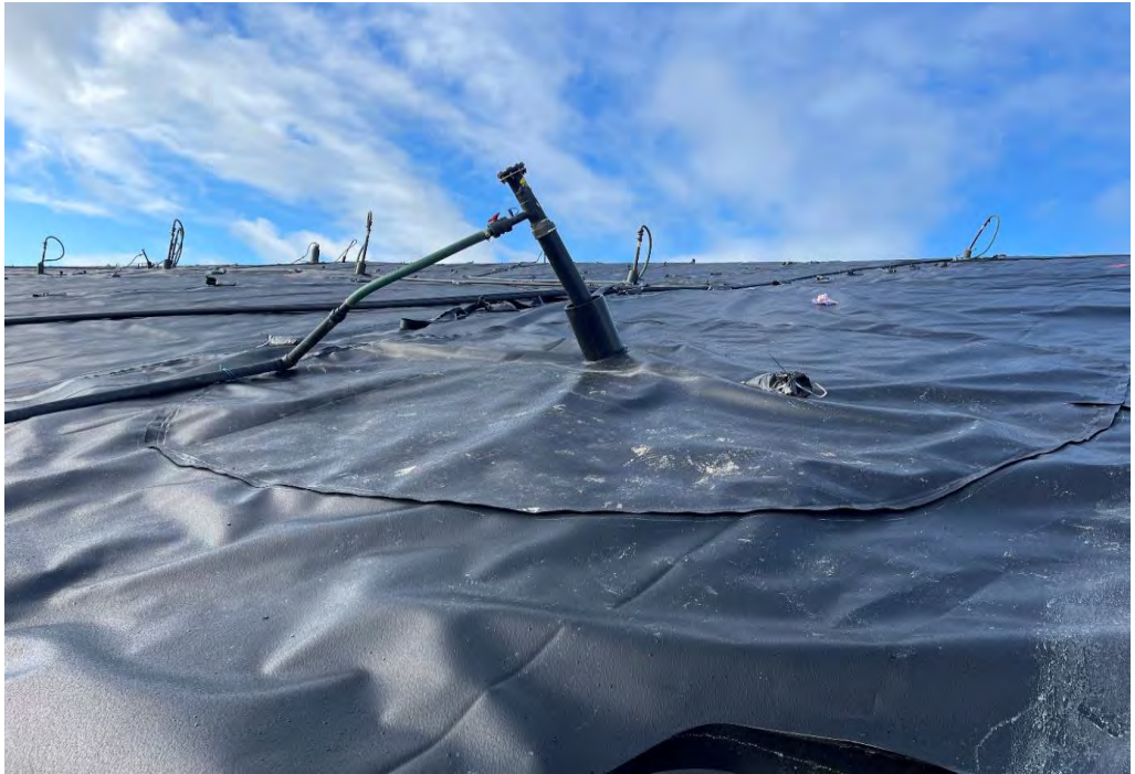
Completed Pipe Boot
