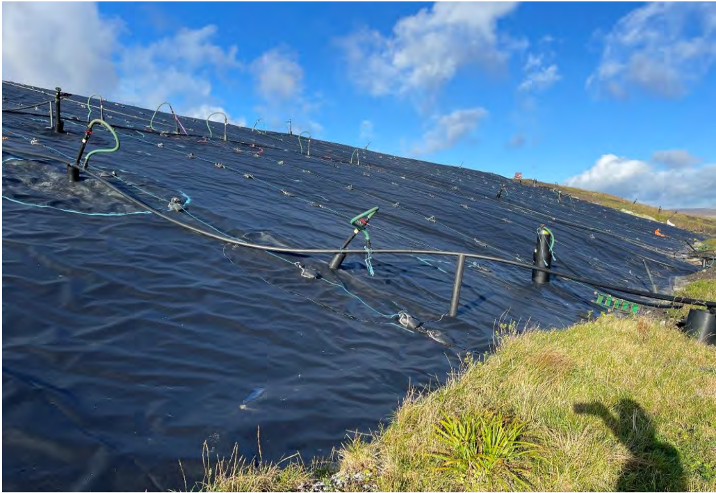
Completed Section of Capping
