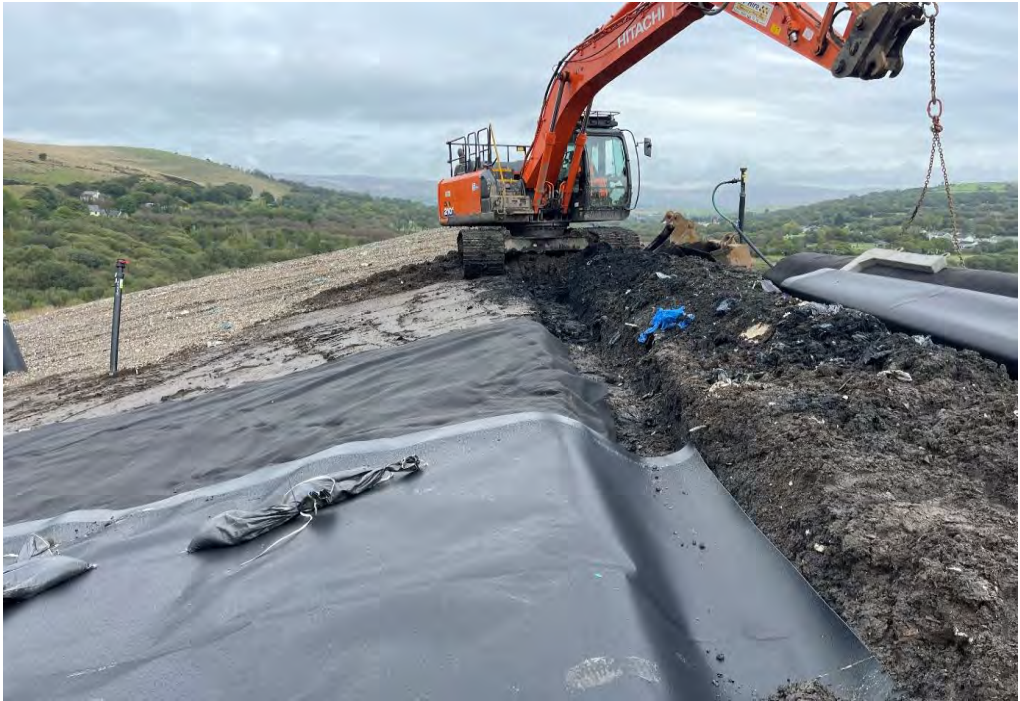
Geomembrane Into Anchor Trench
