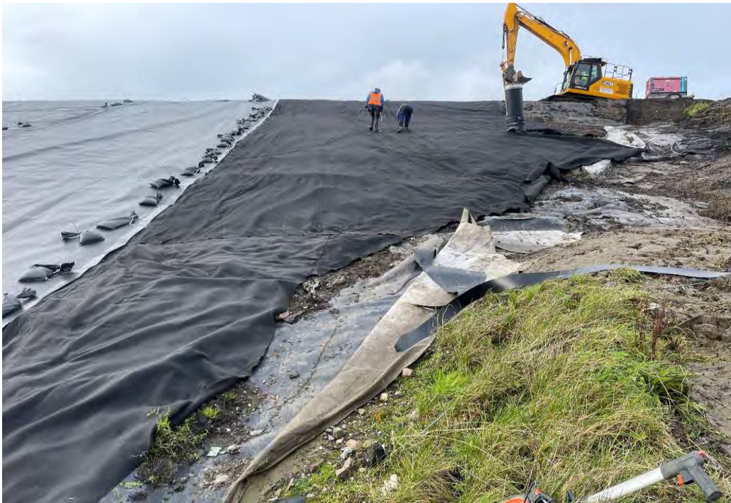
Completed Lower Geotextile Installation
