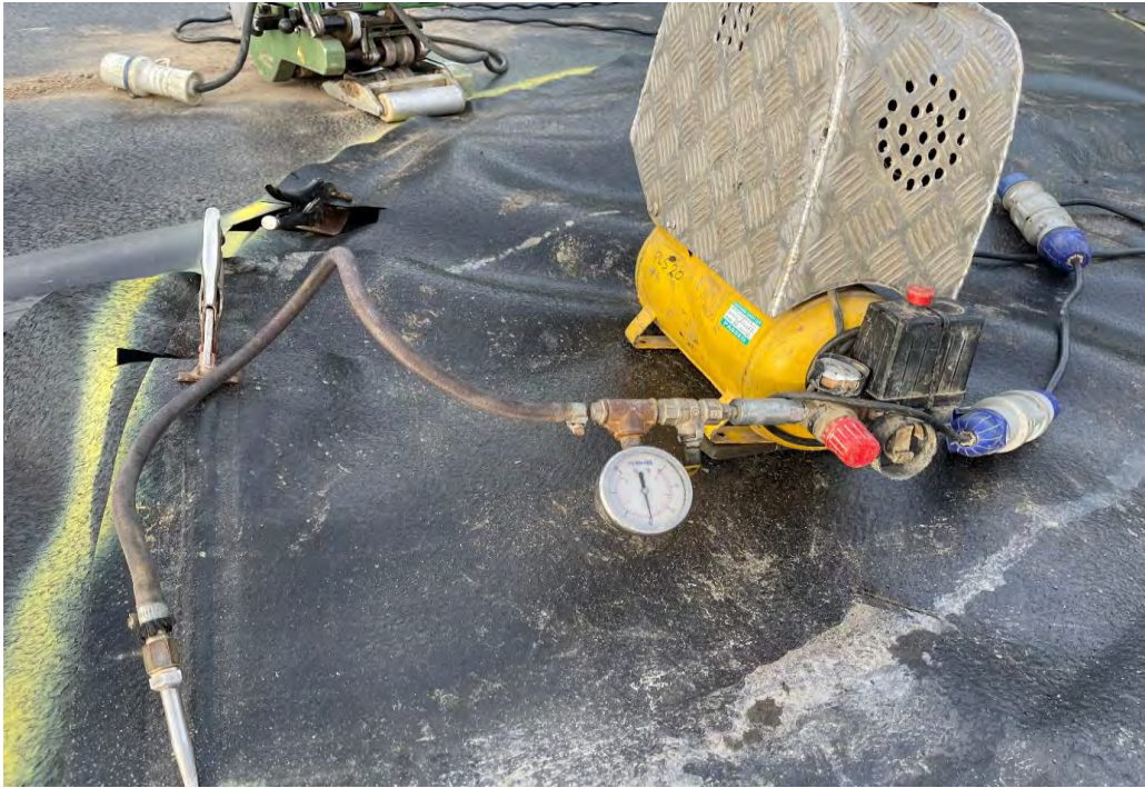
Air Pressure Test in Progress
