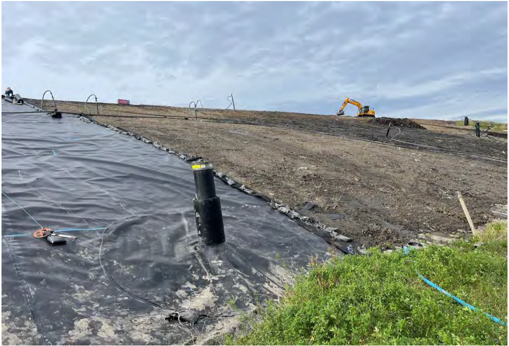
Regulating Layer Preparation
