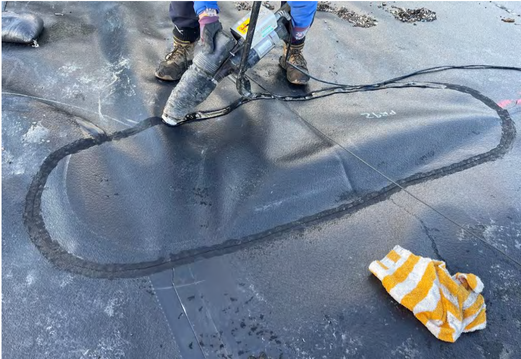
Start of Extrusion Welding
