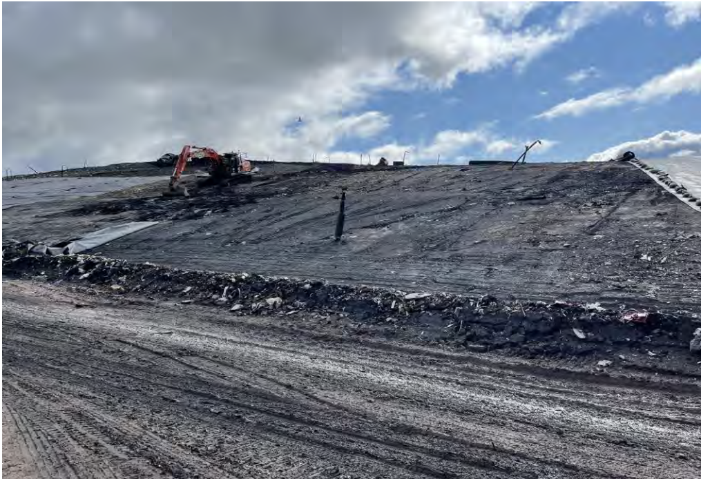
Regulating Layer Preparation
