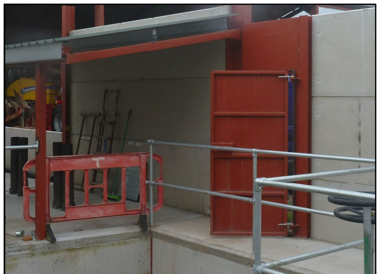
Figure 5. Photograph showing door fitted to containment bund.
