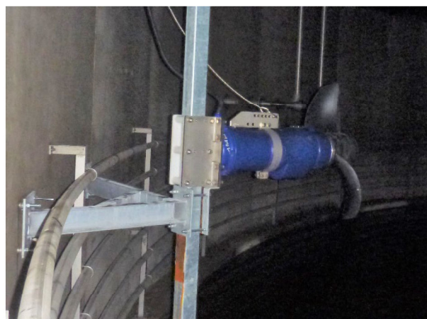
Figures 2 and 3. Photographs showing paddle stirrer (left) and submersible stirrer (above).
