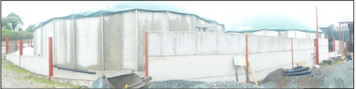
Figure 4. Photograph showing concrete (secondary) containment bund being constructed
