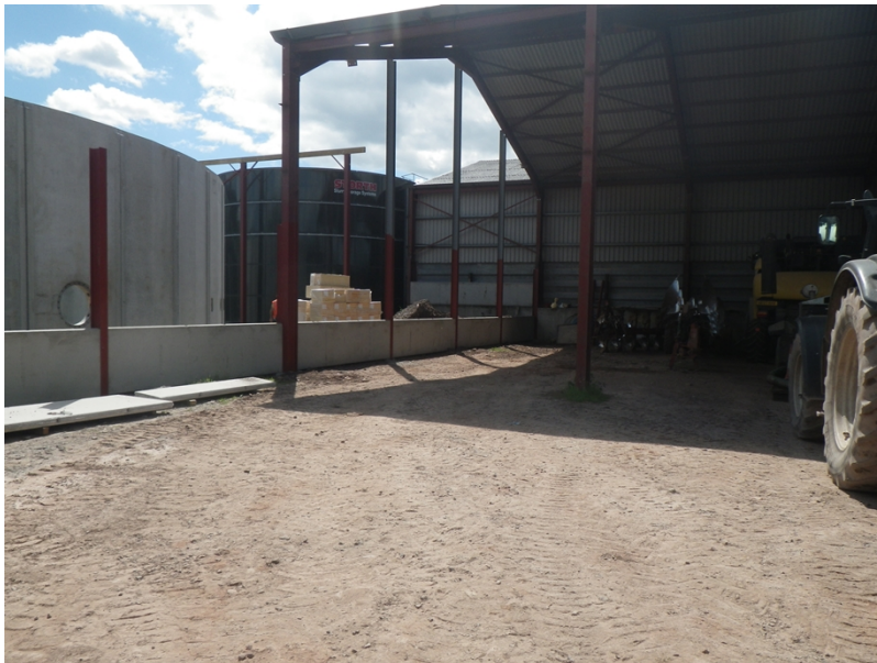
Photo 8: Construction of the new concrete bund
