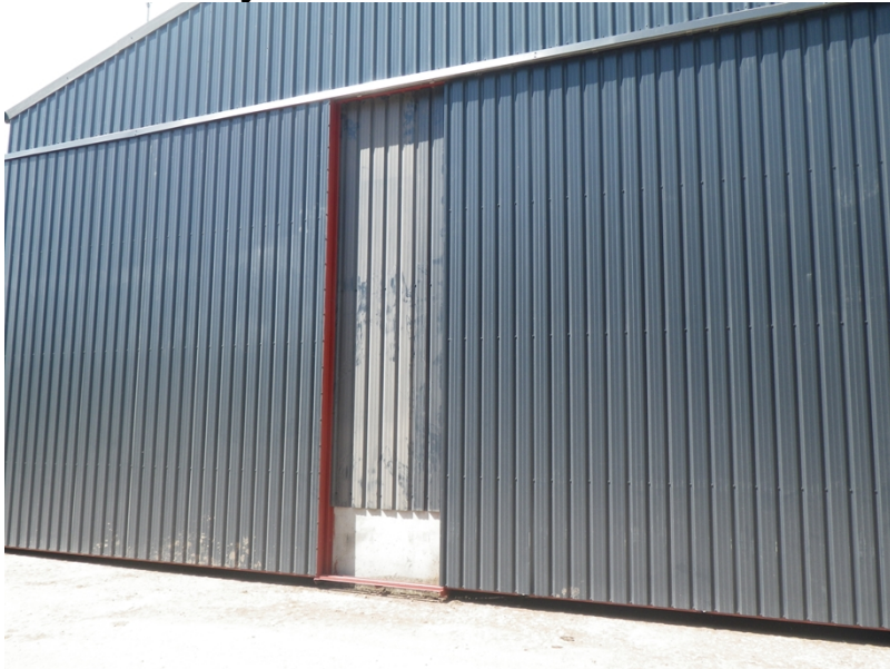
Photo 1: Newly installed doors for odour containment
