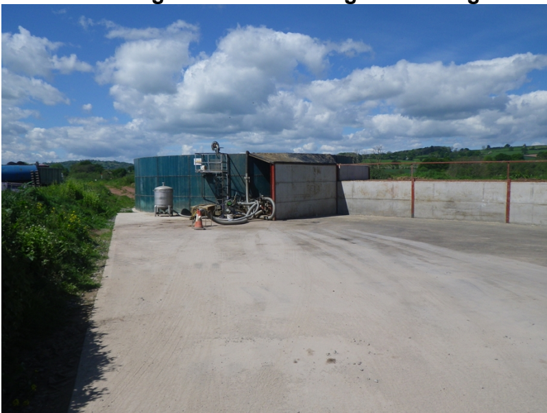
Photo 4: Storage tank and loading / unloading area
