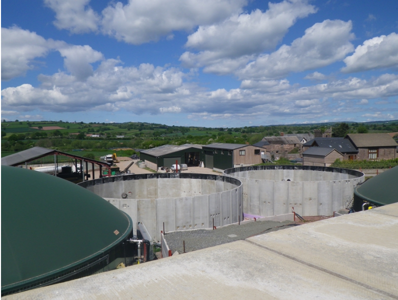
Photo 5: View of the two digesters currently in construction
