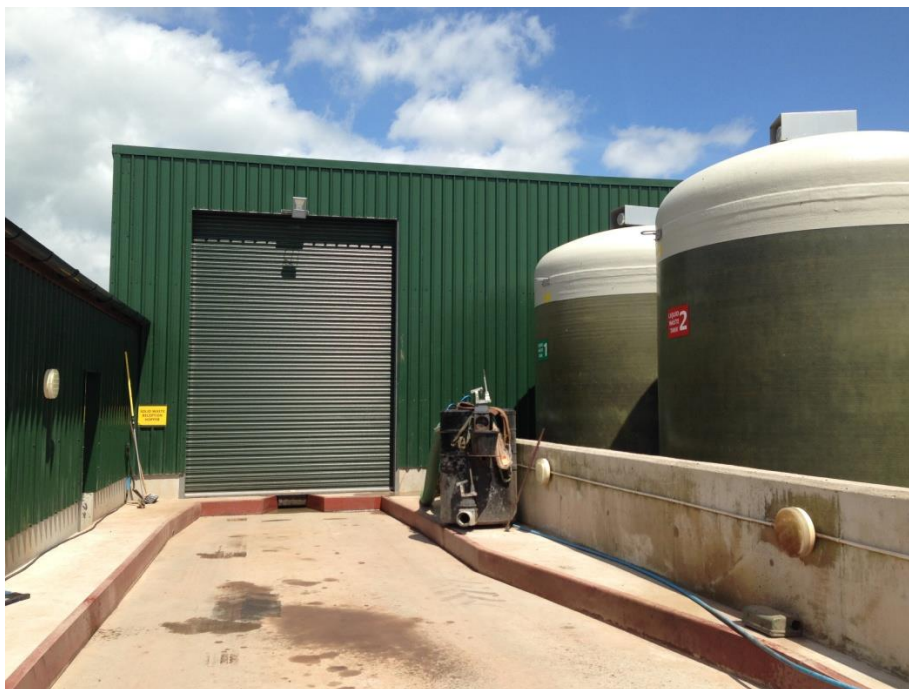
Figure 3.2: Existing ABP Reception and Blood and ABP Fluid Storage Tanks
