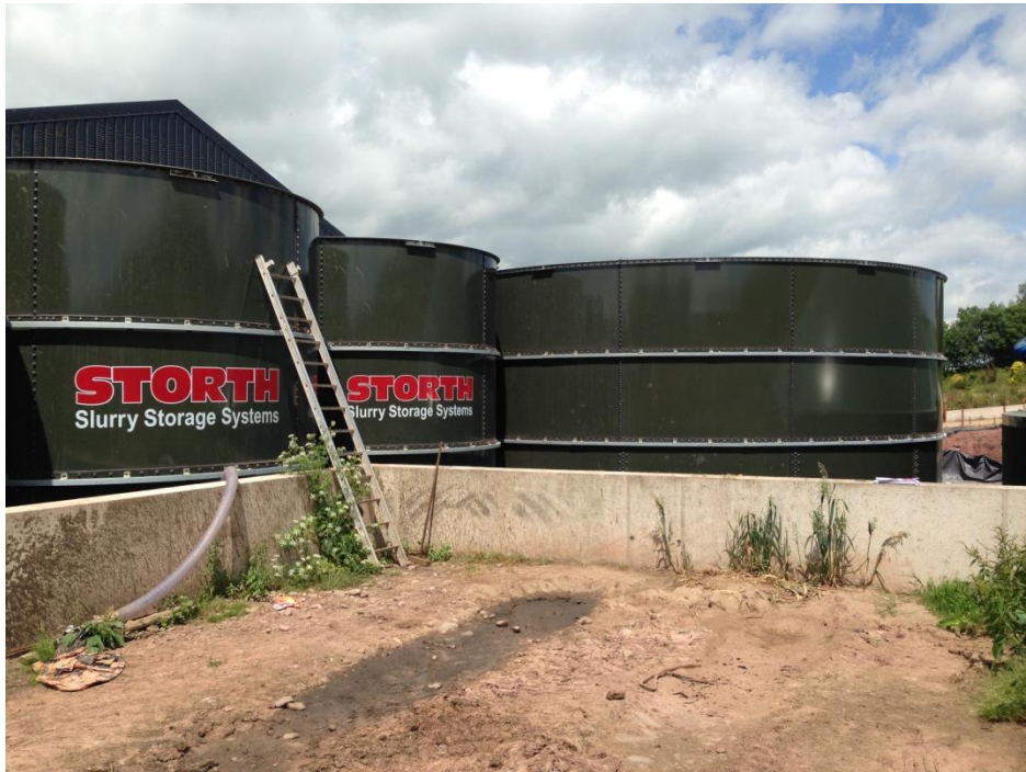
Figure 3.6: Existing Digestate Storage Tanks
