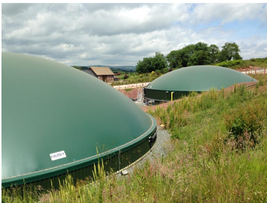
Figure 3.4: Existing Primary and Secondary Digestion Tanks on Site
