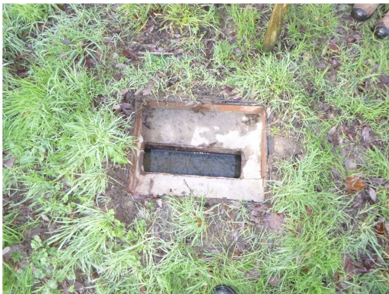
Photograph 3: Final effluent sampling point
