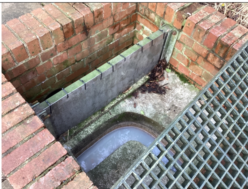
Photograph 2: New grid screen installed at point of overflow
