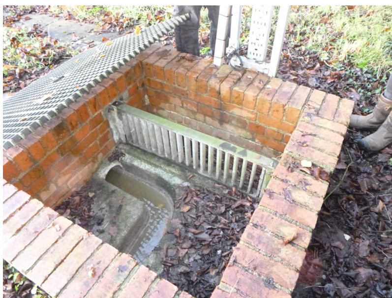
Photograph 1: Clarach STW inlet and overflow bar screen
