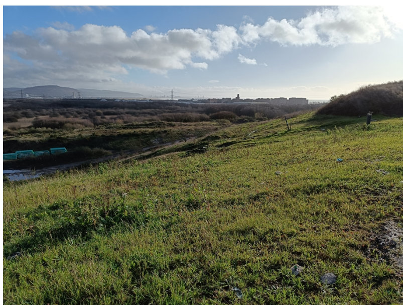
Photo above showing cell 17 with steep flank abutting access road below.
