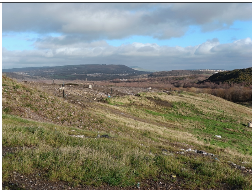
Photo above showing gas wells at top of cell 16 to be capped.
