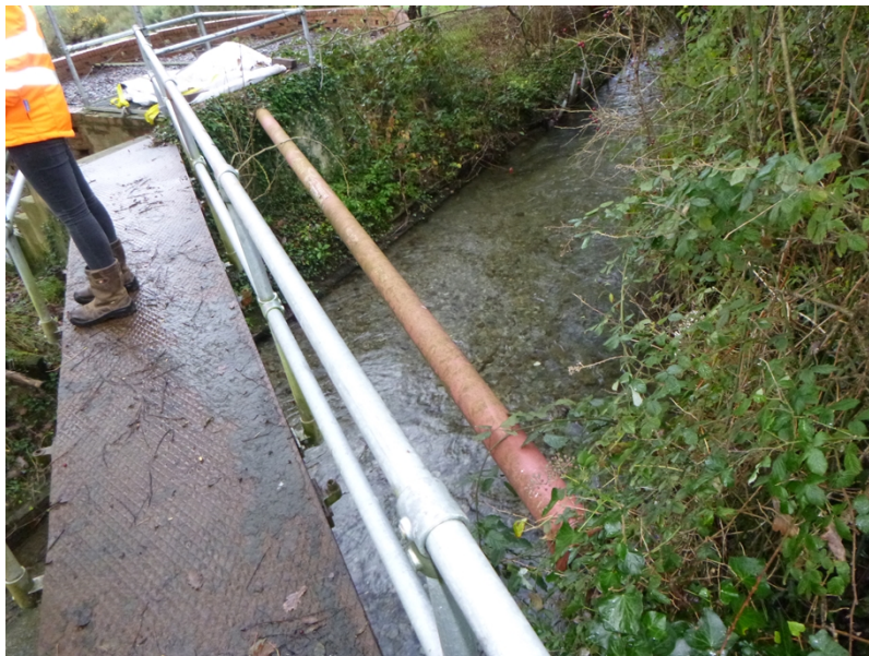
Photograph 3: Raised effluent pipe crossing Afon Melindwr at Capel Bangor WwTW
