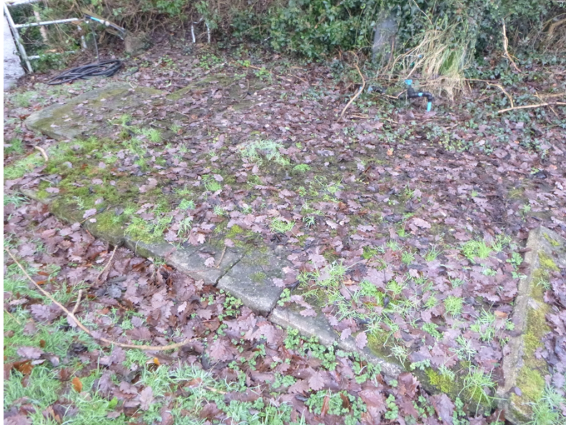
Photograph 2: Below ground septic tanks at Capel Bangor WwTW
