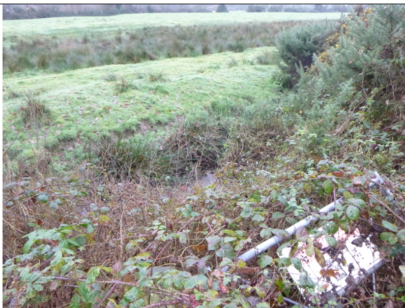
Photograph 7: Final effluent sampling point and outfall into unnamed tributary of the Afon Melindwr
