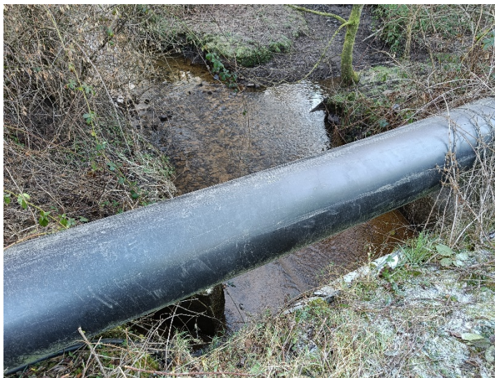
Image 7: Final discharge point to Upper Clydach River
