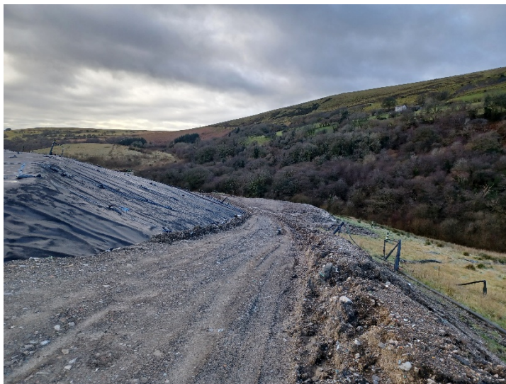
Image 6: Uncapped western flank access road.
