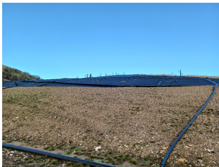
Image 1: Newly capped southern face of Pwllfawatkin Landfill
