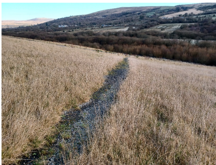
Image 4: French drainage channels installed in restored sections of the landfill.
