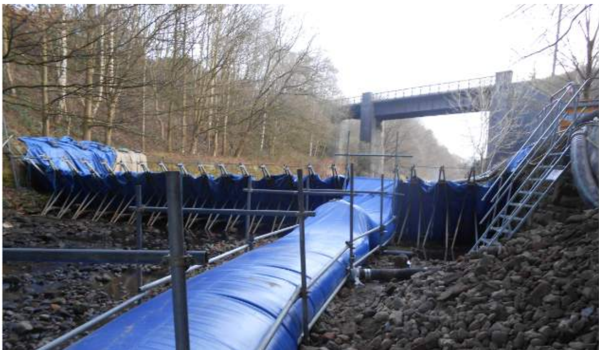
Image of frame dam with flume pipe
