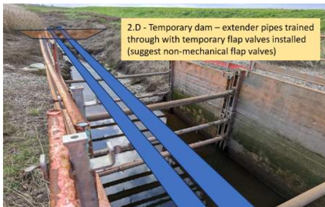
Images showing likely sequence of works under (3), noting temporary dam, not necessary if piles can be driven to specified depths without requirement for struts
