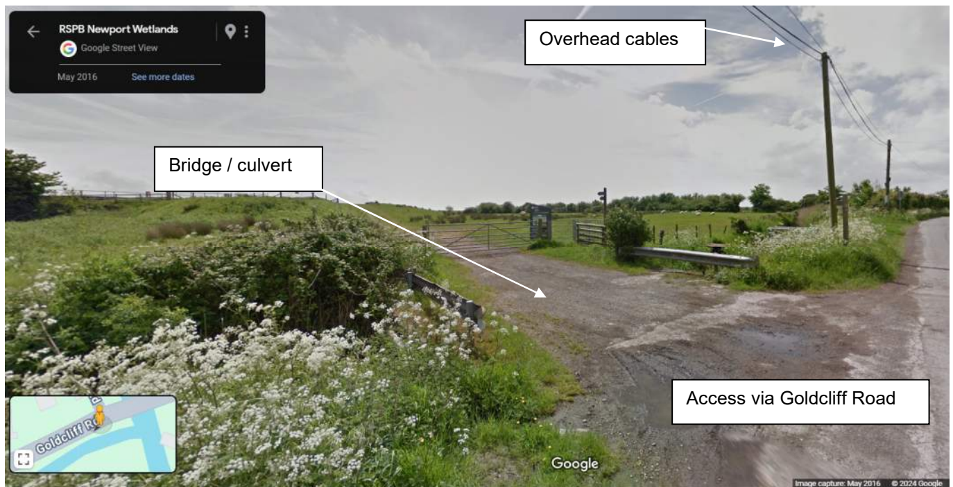
Image showing access to site via Goldcliff Road, noting bridge / culvert crossing and overhead cables.
