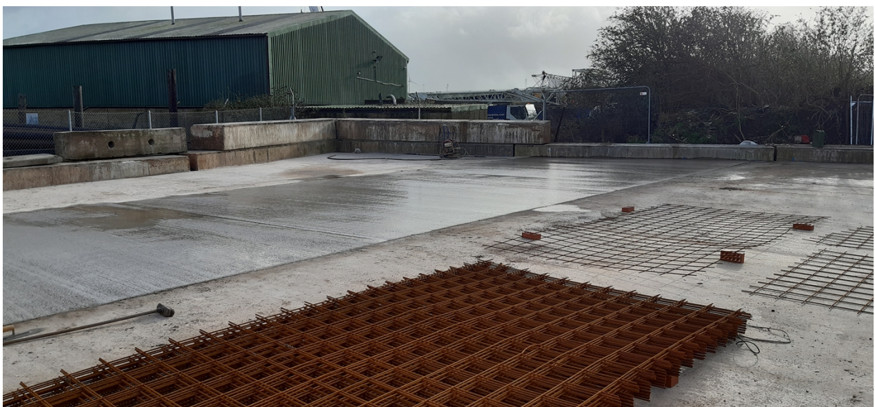
Photo 2 - Site infrastructure in good condition with improvement works ongoing
