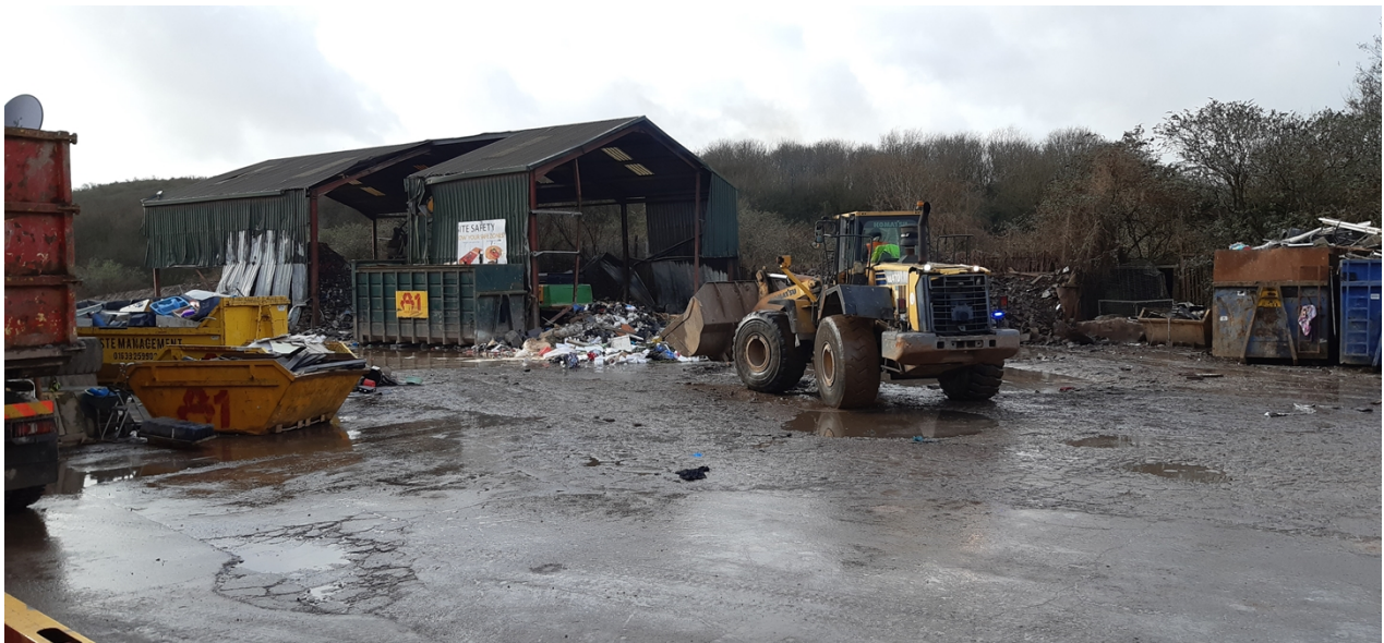
Photo 1 - Site infrastructure in good condition with improvement works ongoing
