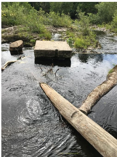
Plate 4-11. Structure in channel at weir (one end of where stoplogs can be inserted to dry up channel to canal for when that is maintained)
