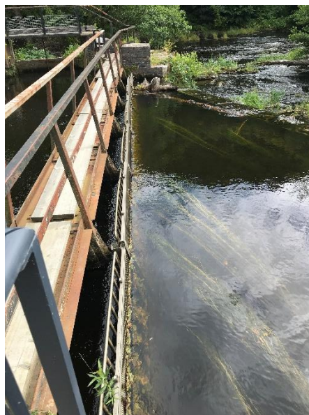
Plate 4-12. Screens at entrance to canal feeder stream
