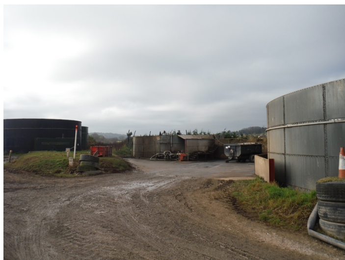
Permitted area BB3099CG - clamp & store in centre of photograph, 12/01/2024
