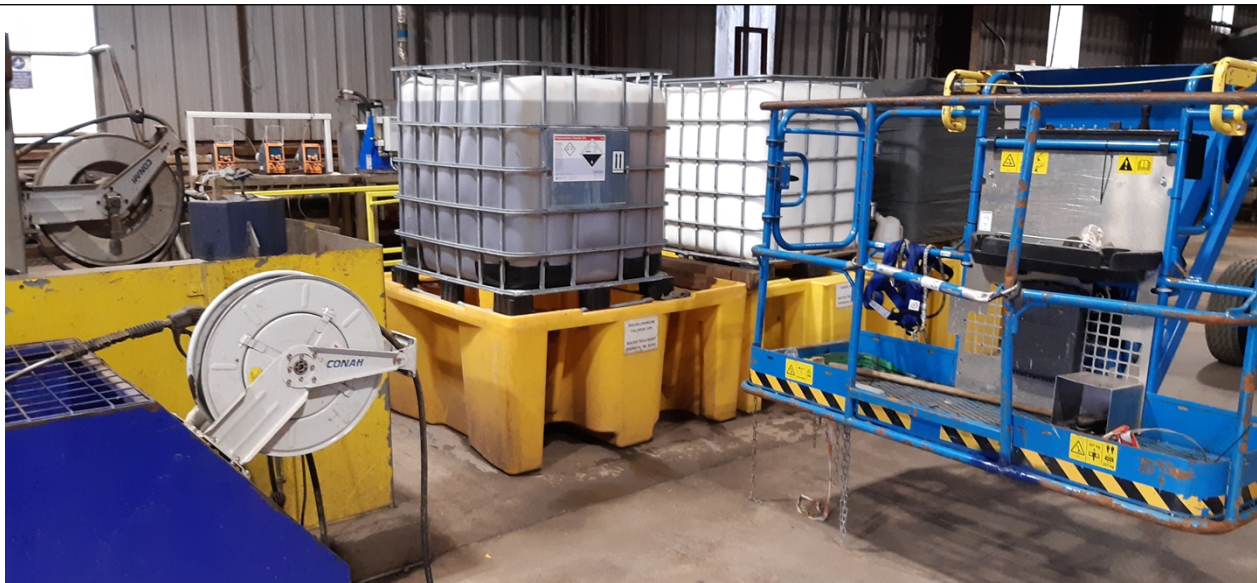
Photo 5 - Secondary containment bund for liquid storage
