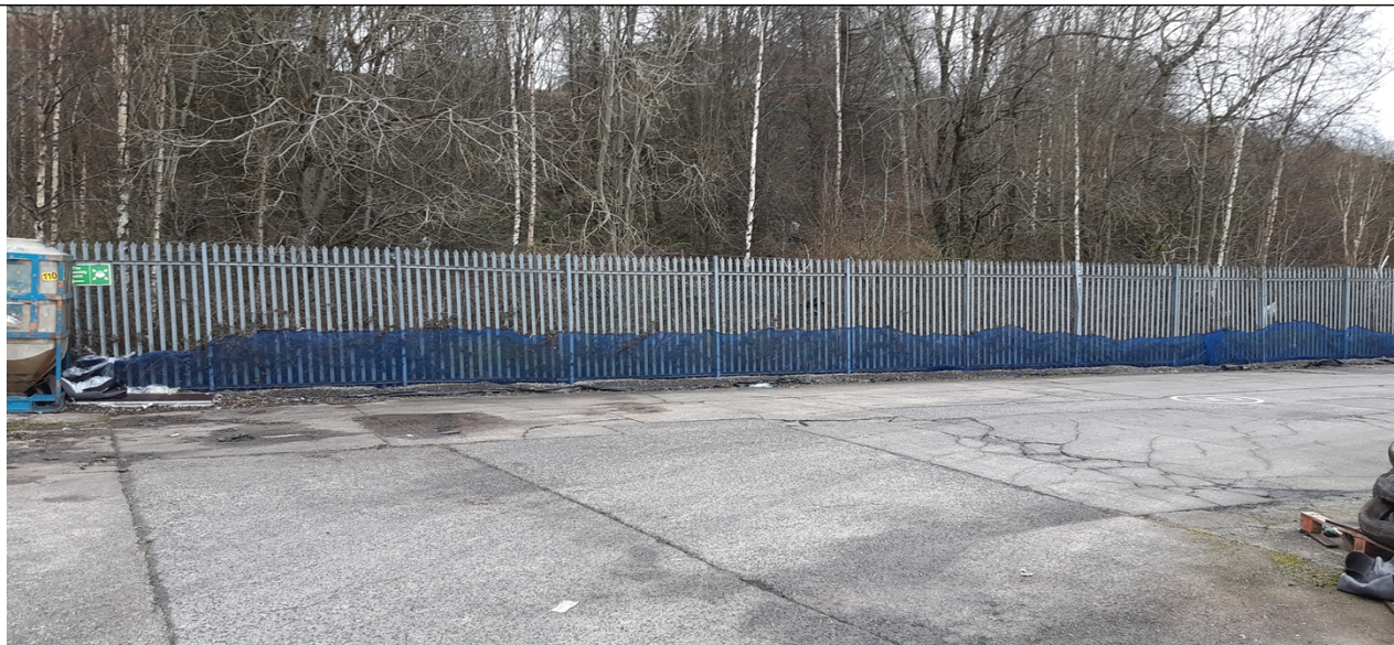
Photo 3 - Netting around perimeter of site preventing litter escaping site
