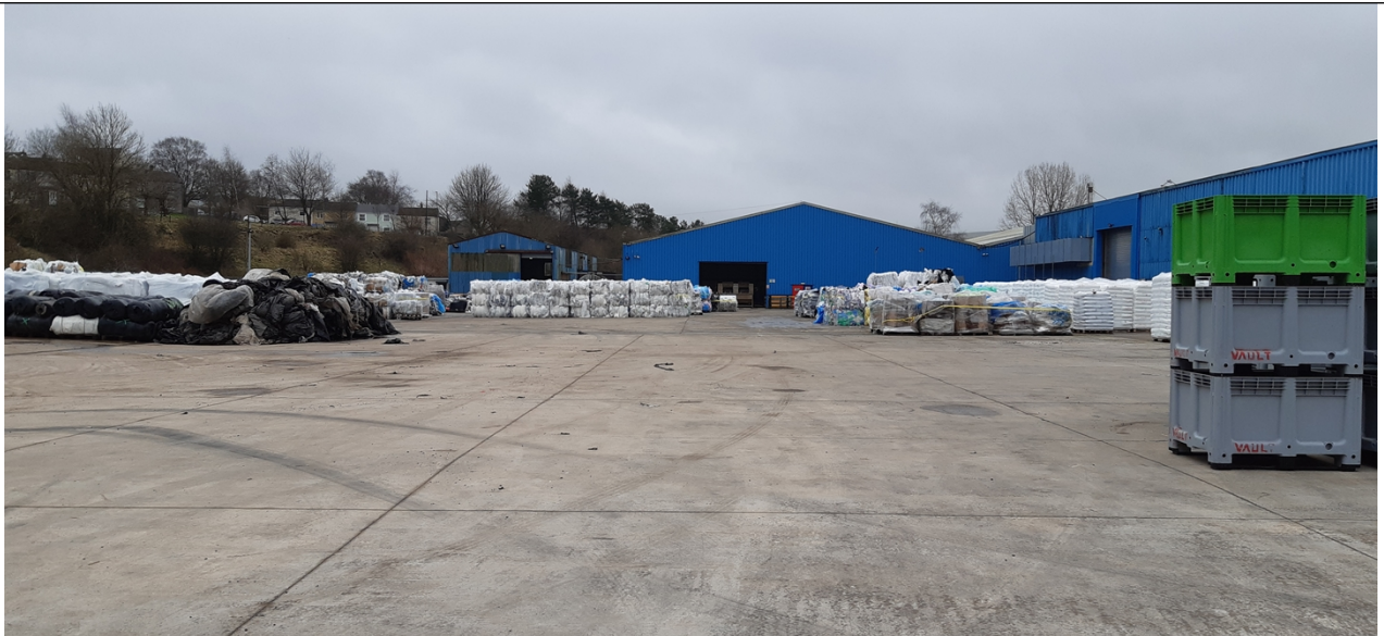
Photo 1 - Good housekeeping practices located in yard outside and on site in general
