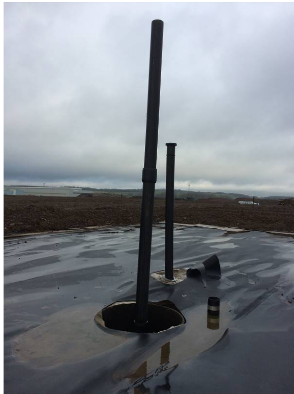
Plate 4. Construction of Gas Vents through Capping Systems
