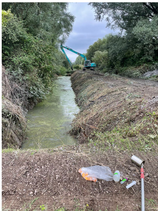
Plate 6-4 Ditch maintenance during August 2021 sampling upstream of sample point SW1
