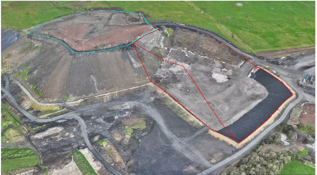
Figure 1-2 Cell 8 Works Area
