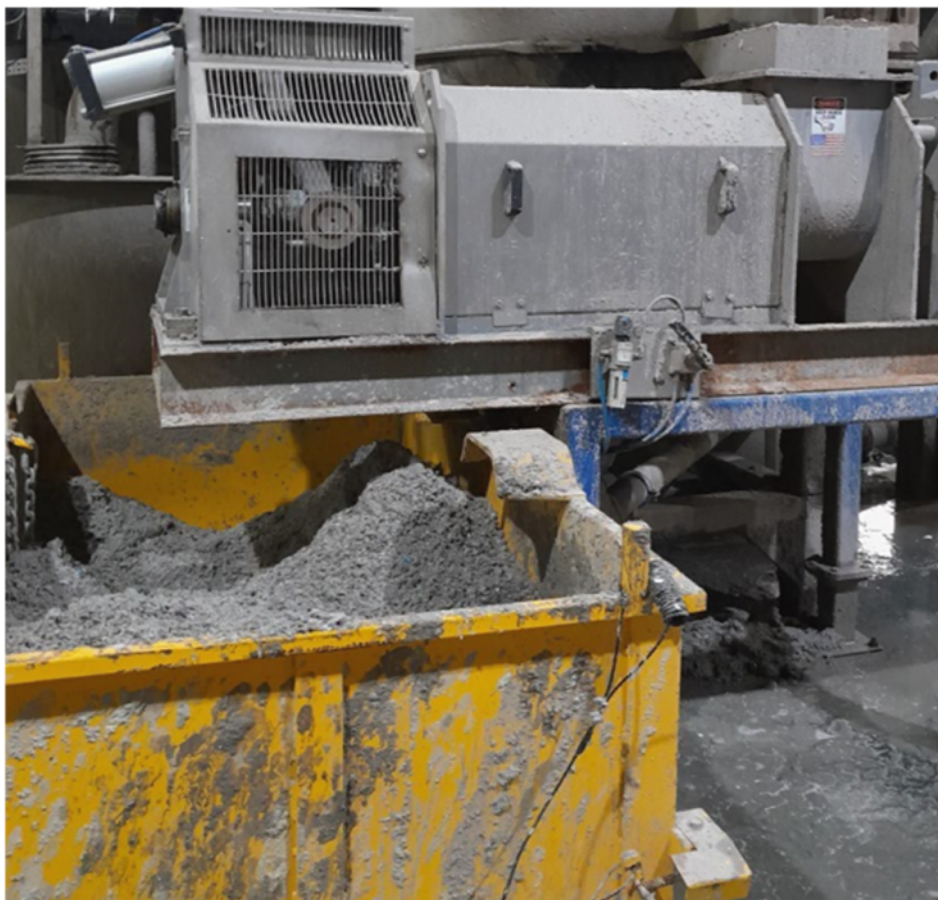
Image 2 - Showing the de-watering screw operating to full capacity
