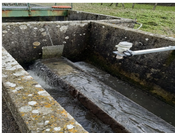
Inlet Discharging to storm tank
