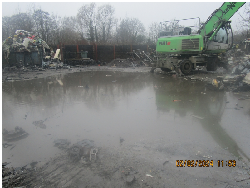
photo 1 - pooling of water on site
