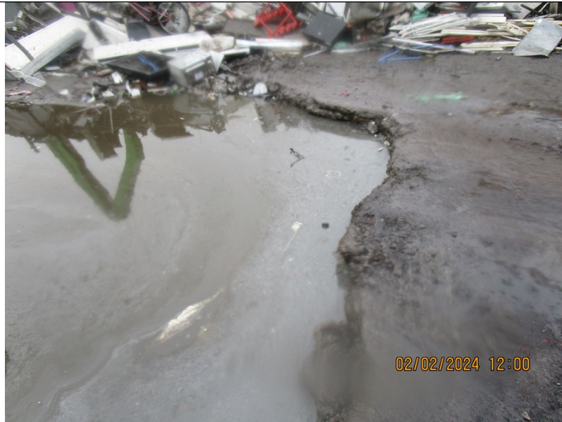
Photo 3 badly damaged concrete
